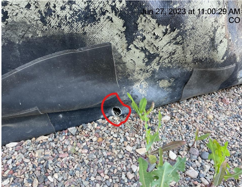
Photo # 1665 From Inspection 708900897 conducted on 06/27/2023 Hole in liner/liner needs maintenance
