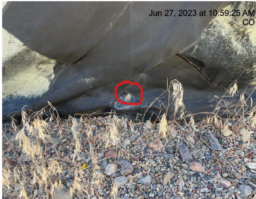
Photo # 2069 From Inspection 708900897 conducted on 06/27/2023 Hole in liner/liner needs maintenance
