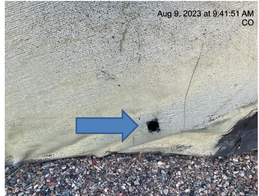
Photo # 5467 Hole in liner/liner needs maintenance
