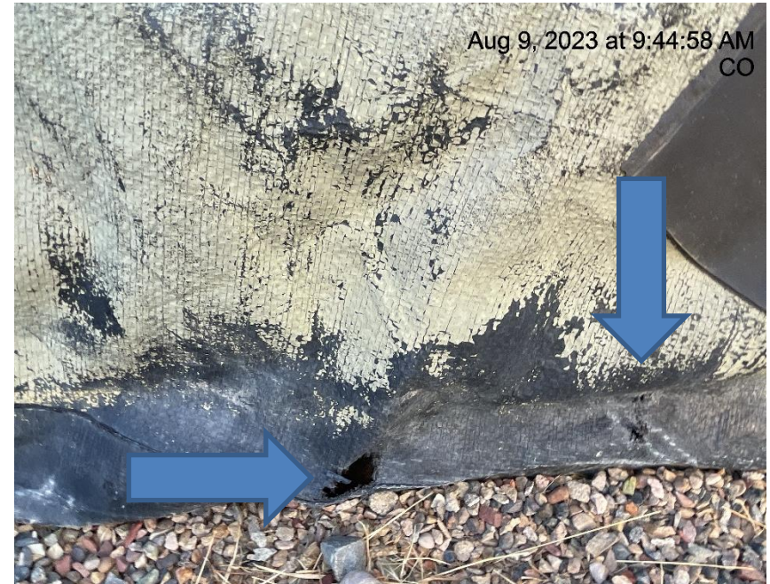
Photo # 5520 Holes in liner/liner needs maintenance
