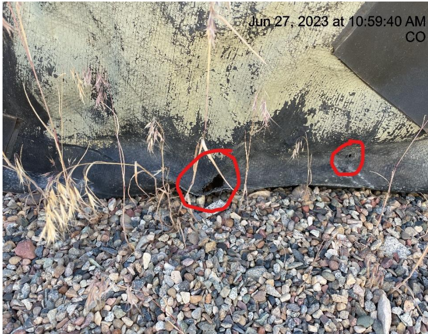
Photo # 2071 From Inspection 708900897 conducted on 06/27/2023 Holes in liner/liner needs maintenance
