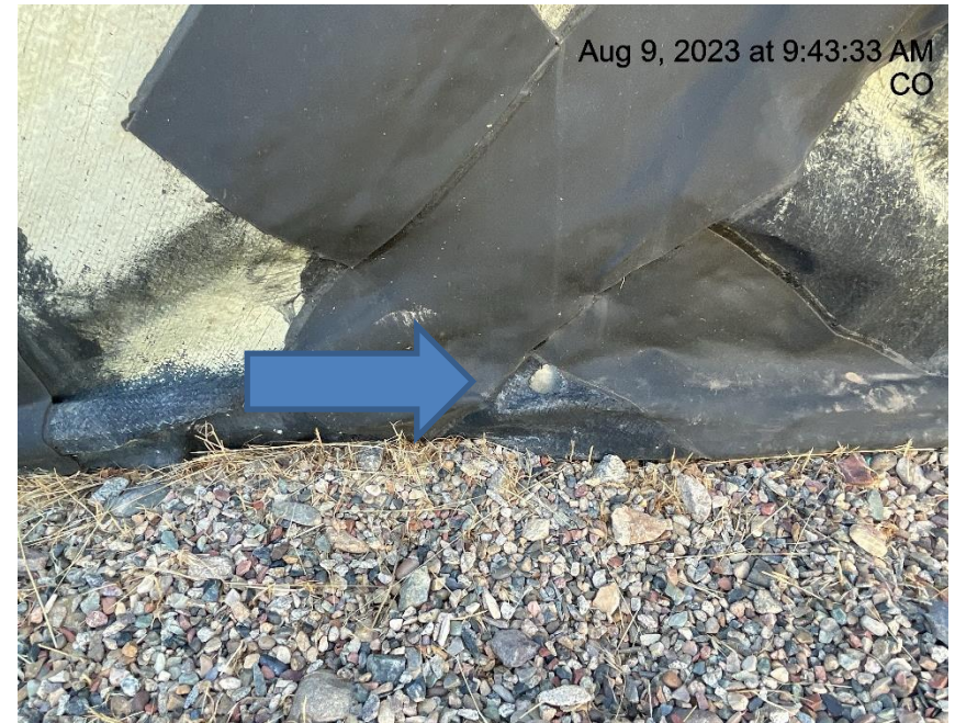
Photo # 5470 Hole in liner/liner needs maintenance
