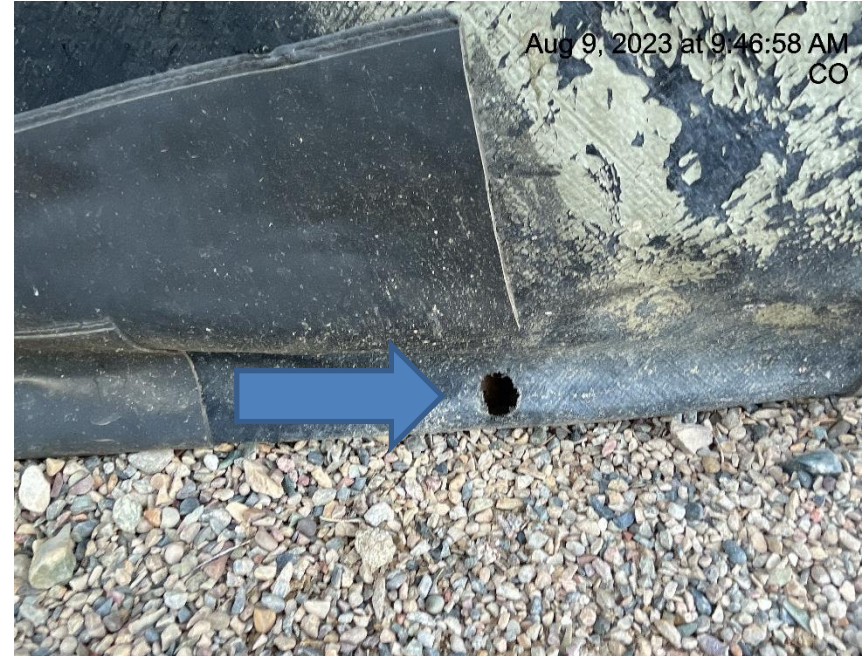
Photo # 5523 Hole in liner/liner needs maintenance
