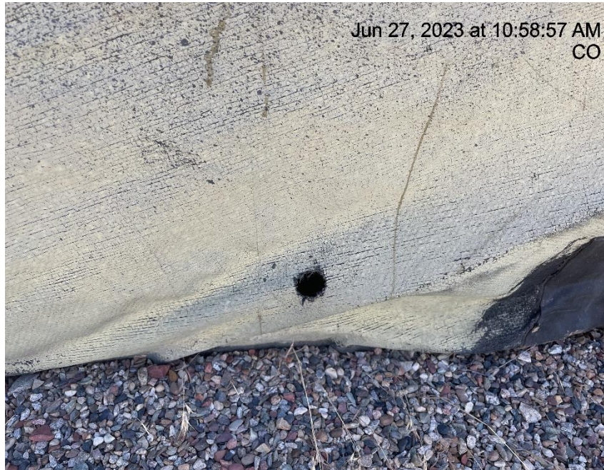
Photo # 2067 From Inspection 708900897 conducted on 06/27/2023 Hole in liner/liner needs maintenance
