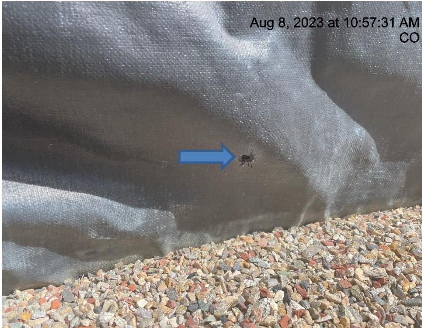
Photo # 5266 Hole in containment liner/liner needs maintenance
