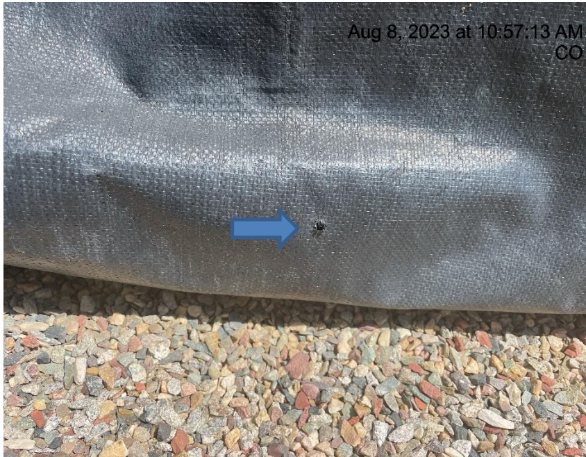
Photo # 5264 Hole in containment liner/liner needs maintenance
