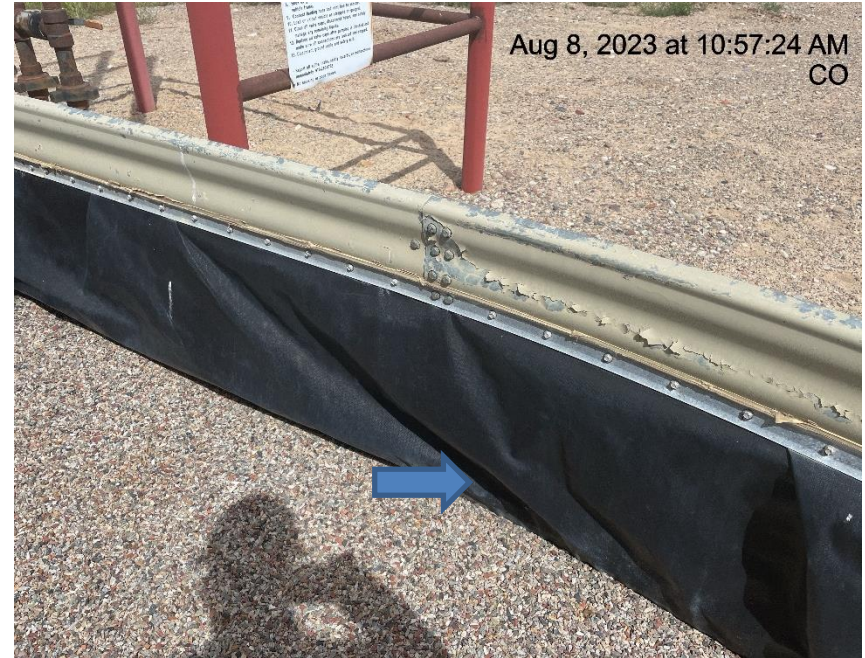
Photo # 5265 Hole in containment liner/liner needs maintenance
