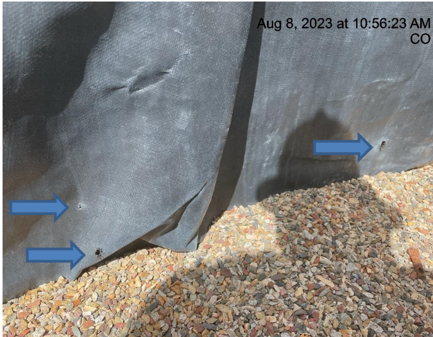
Photo # 5261 Holes in containment liner/liner needs maintenance
