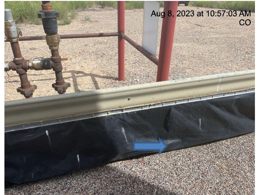
Photo # 5263 Hole in containment liner/liner needs maintenance
