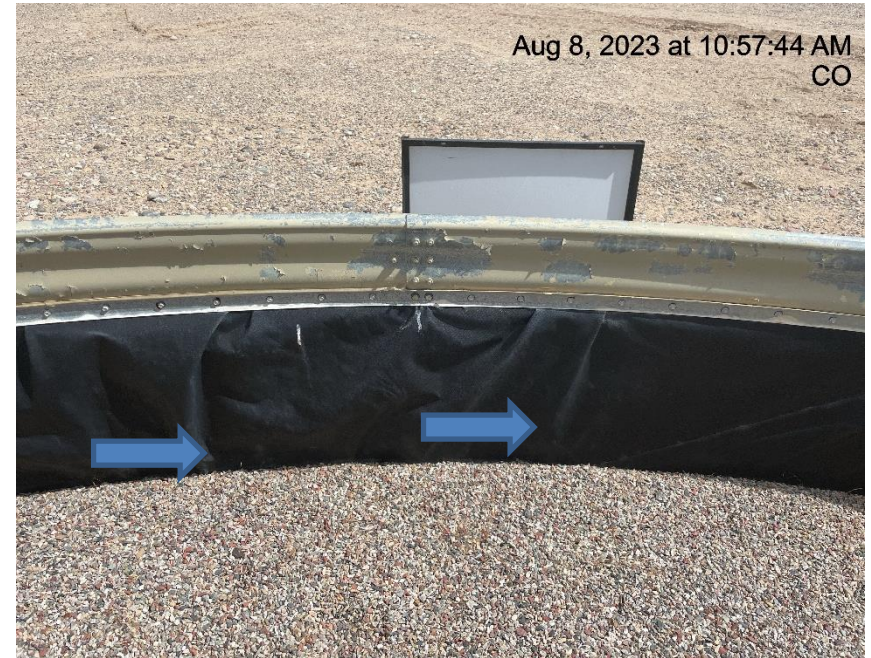
Photo # 5268 Holes in containment liner/liner needs maintenance
