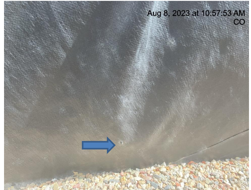
Photo # 5279 Hole in containment liner/liner needs maintenance
