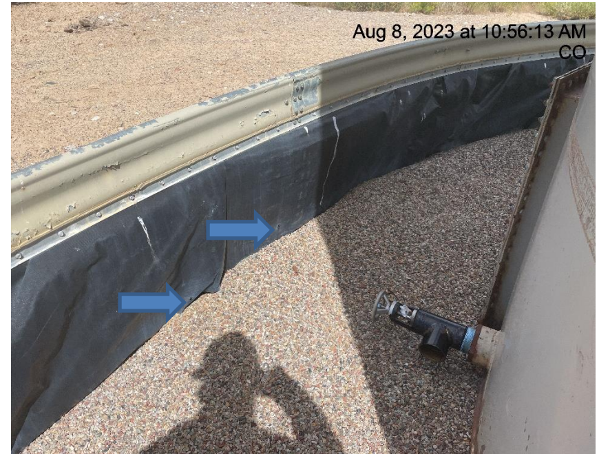
Photo # 5260 Holes in containment liner/liner needs maintenance
