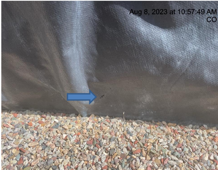
Photo # 5269 Hole in containment liner/liner needs maintenance
