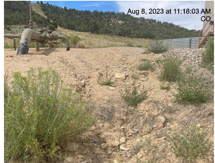
Photo # 5307 Erosion & transport of sediment (East edge of location near tank battery)
