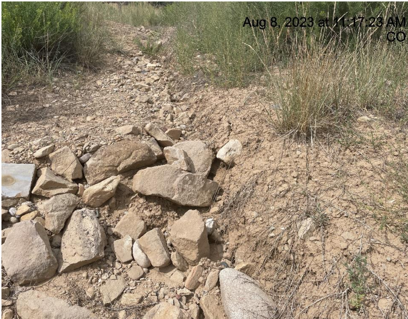
Photo # 5303 Rip Rap Run/BMP's need maintenance (East edge of location near tank battery)
