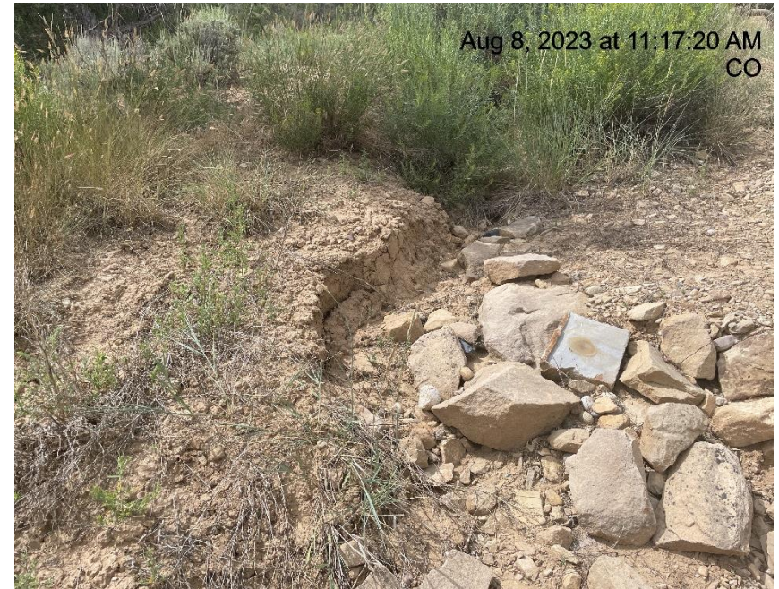
Photo # 5302 Rip Rap Run/BMP's need maintenance (East edge of location near tank battery)
