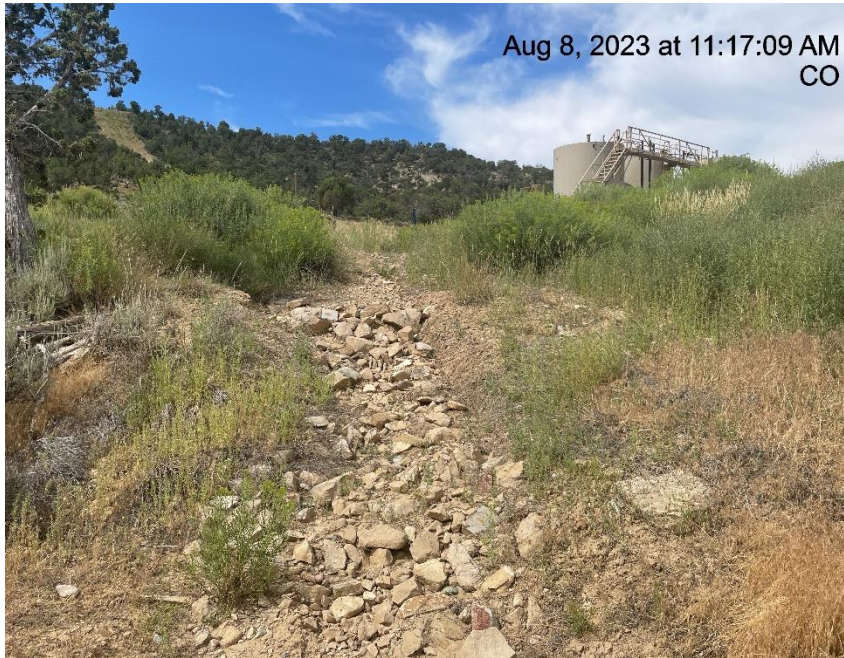
Photo # 5301 Rip Rap Run/BMP's need maintenance (East edge of location near tank battery)
