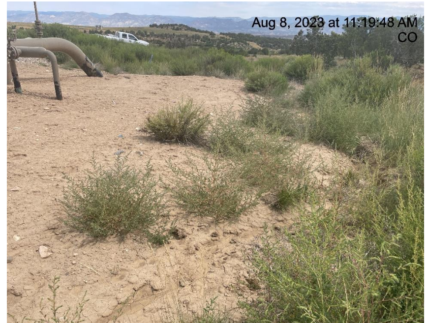
Photo # 5312 Erosion & transport of sediment (East edge of location near tank battery)
