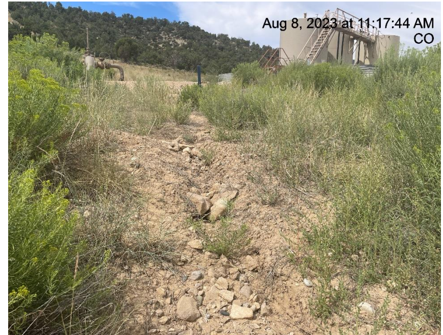
Photo # 5304 Erosion & transport of sediment/BMP's need maintenance (East edge of location near tank battery)
