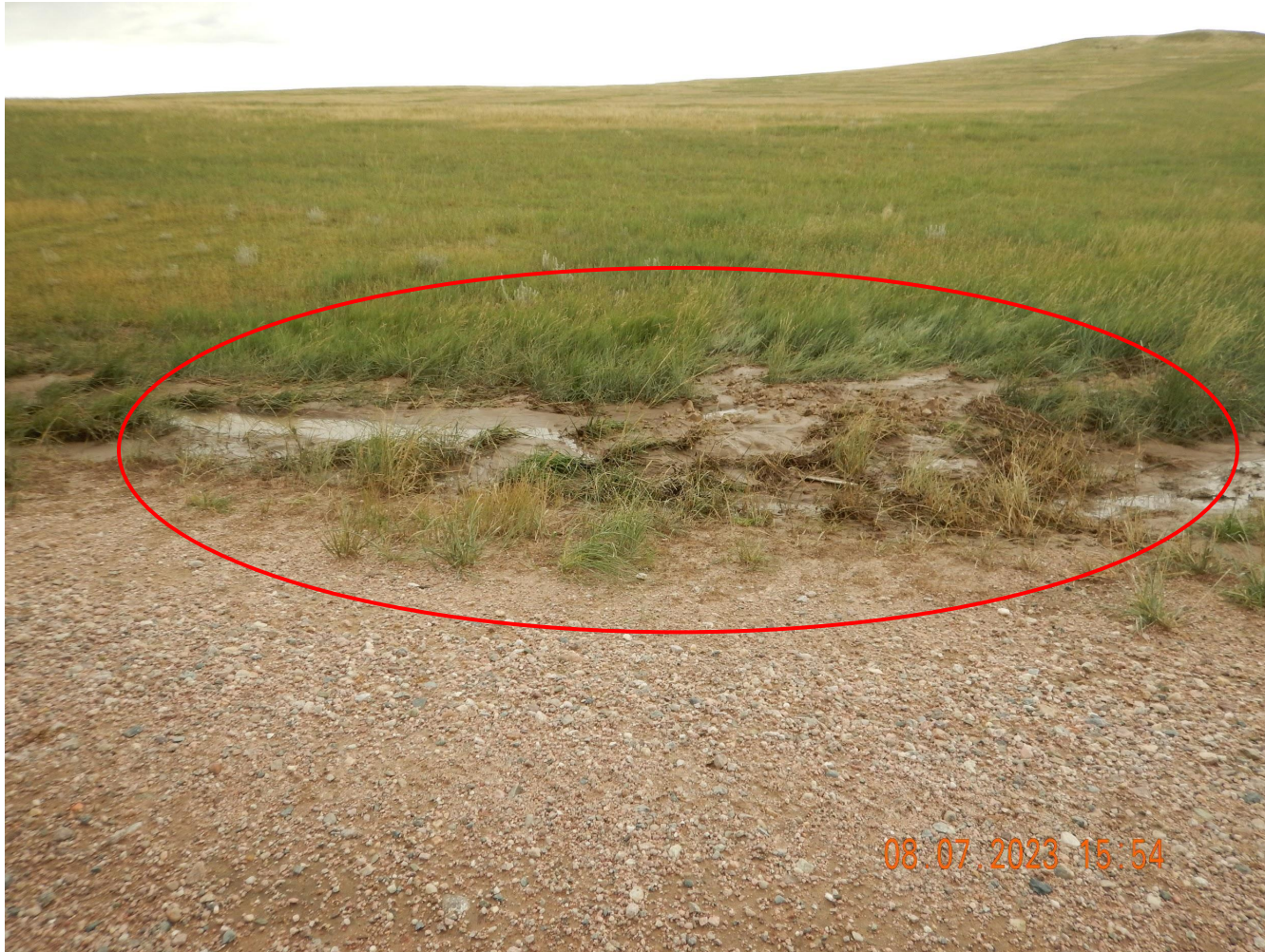
Photo 9. Photo illustrates sediment accumulation at the bottom of the slope from unstabilized ditch areas along the access road previously shown in Photos 7-8.
