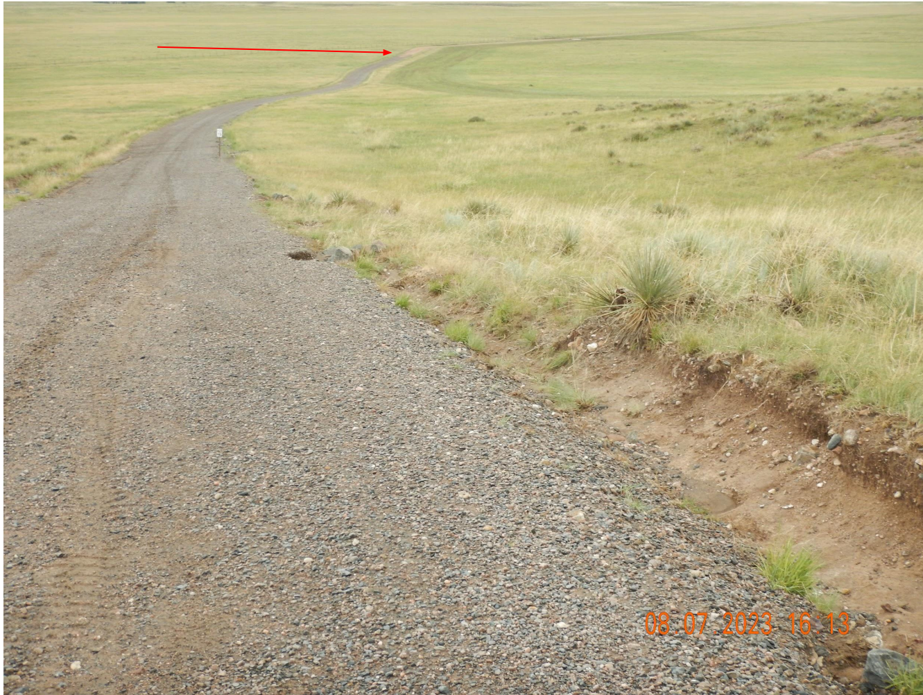
Photo 13. Photo illustrates the Operator imported new road base (lighter color) but stopped around the 2 mile marker. When Staff traveled on this road back on July 14th, dust was minimized along the new import but dust increased once on the darker road base sections. Operator has not completed dust mitigation work.
