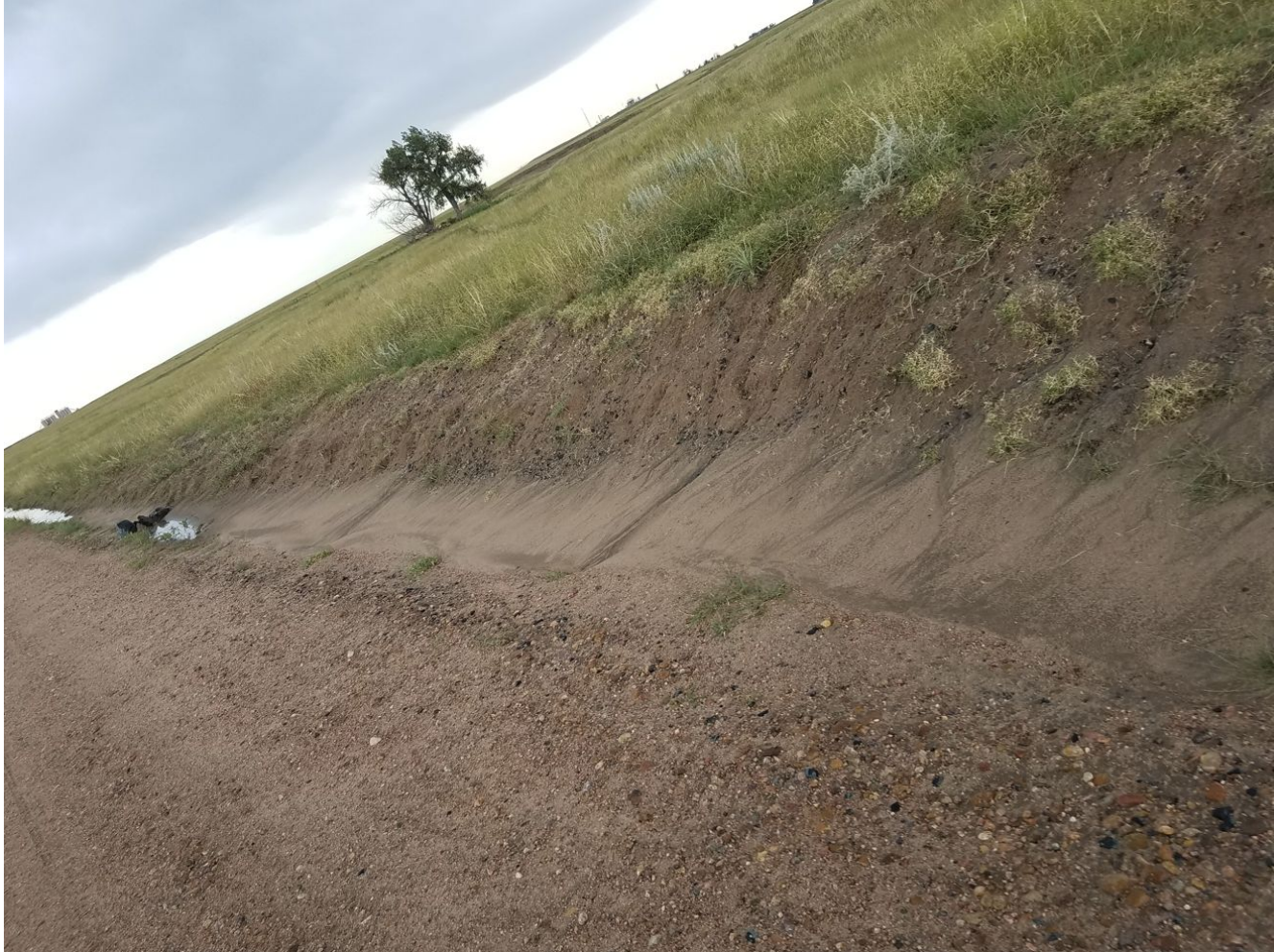
Photo 18. Photo taken east of Geary Creek, facing Southeast. Photo illustrates a section of cut slope that was disturbed during snow removal. Operator has failed to reclaim and stabilize the cut slope that continues to erode into Geary Creek.
