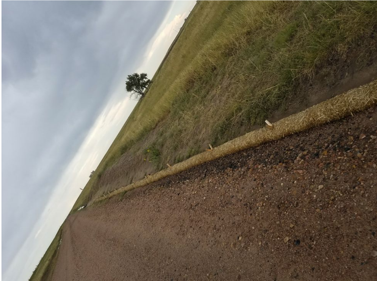
Photo 16. Photo taken east of Geary Creek, facing East. Photo illustrates an improperly installed straw wattle that appears to be for a section of cut slope along the access road. Operator still has not installed sufficient BMPs to minimize erosion into Geary Creek.
