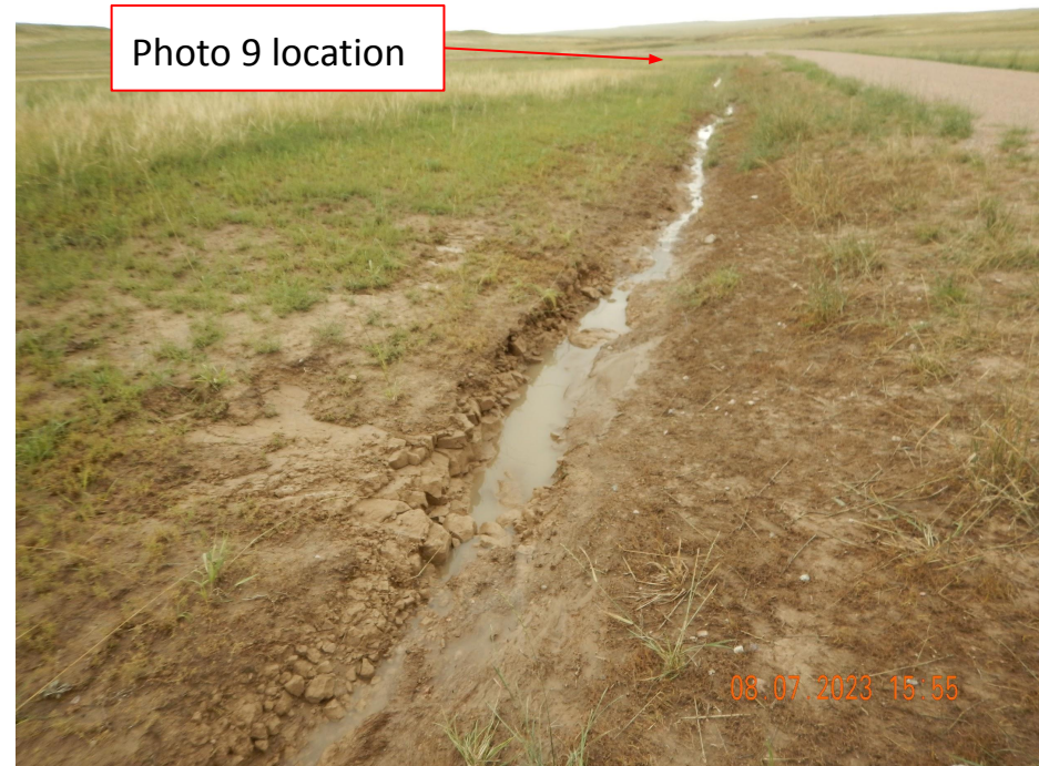
Photo 8. Photo taken from the previous photo location, facing the opposite direction. Again, photo illustrates weed management issues and stormwater erosion issues.
