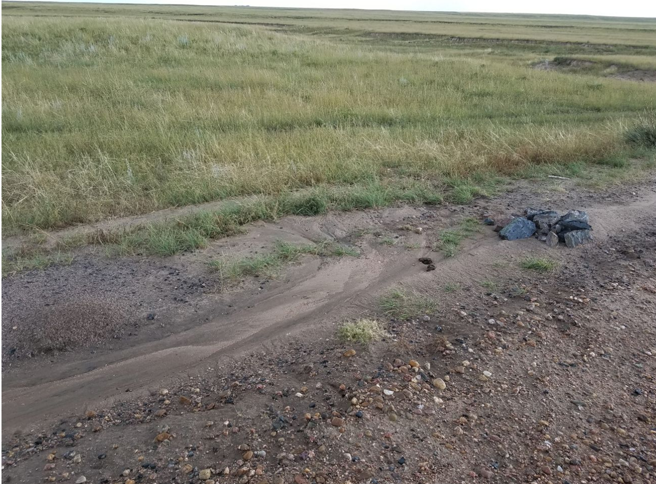
Photo 17. Photo taken east of Geary Creek, facing South. Photo illustrates a check dam BMP that is not in proper functioning condition and Operator still has not installed sufficient BMPs to minimize erosion into Geary Creek. This BMP has remains in the same configuration since the previous inspection in June.
