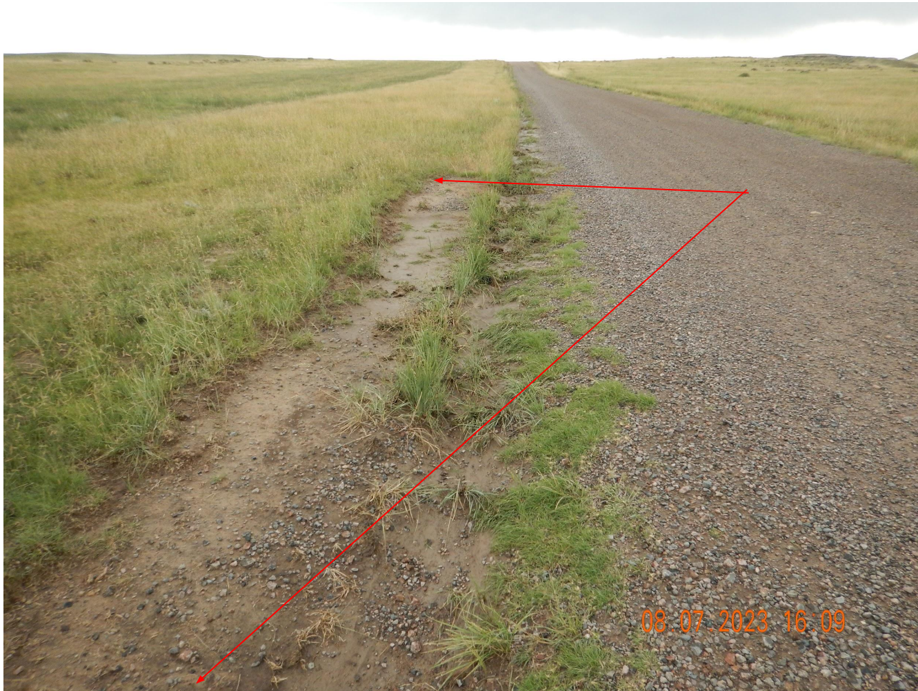
Photo 15. Photo illustrates another section which is off the lease road that the Operator disturbed during snow removal. In this example, Operator scrapped off the topsoil from the area and has failed to reclaim sections like these throughout the access road. These sections are being left unstabilized, causing erosion and weed establishment is occurring along these sections.
