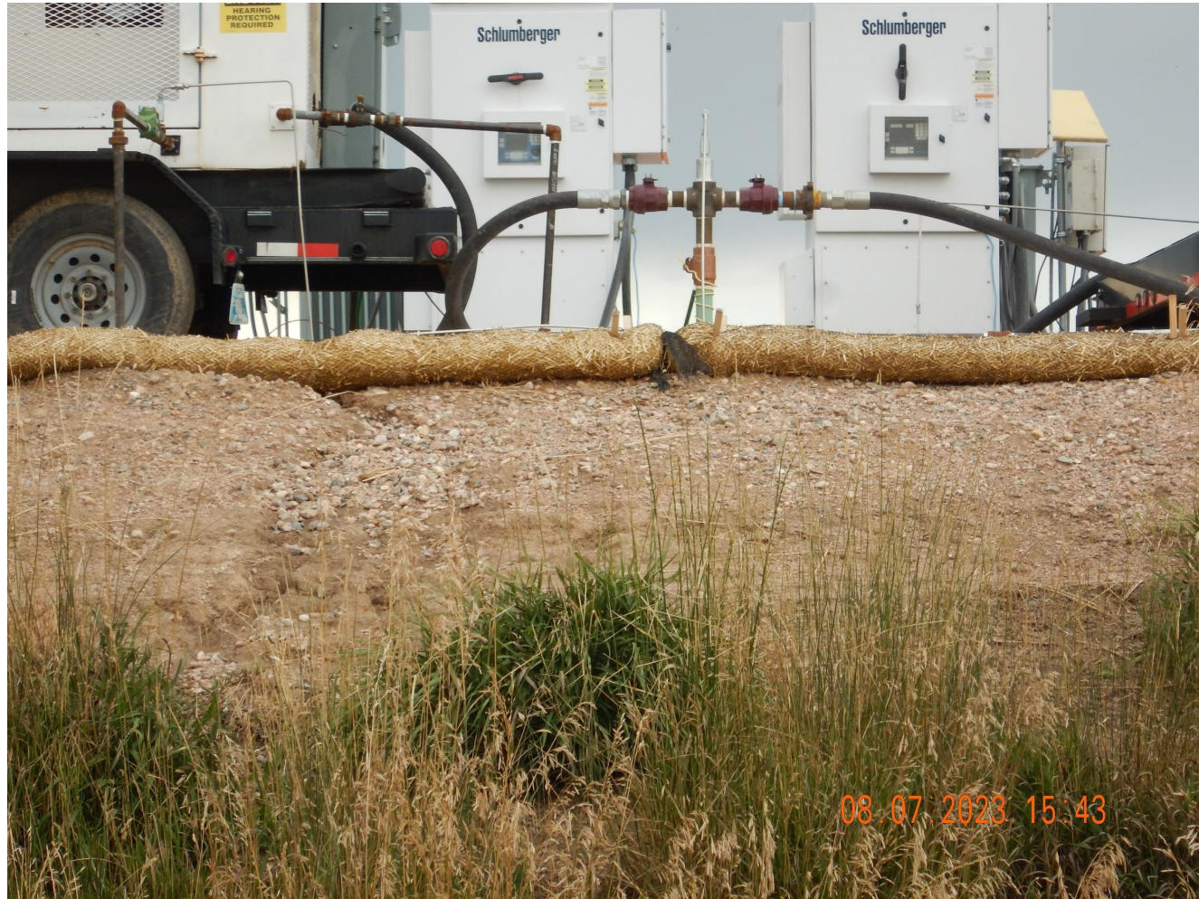
Photo 20. Photo taken along the southern location, facing North. Photo illustrates the BMP has not been properly installed (has not been trenched or proper overlap) and stormwater is undermining the BMP.
