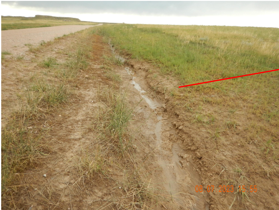
Photo 7. Photo taken from a portion of the access road, illustrating weed management and stormwater erosion. Weed growth is observed beyond the red line; however, weeds appear to be sprayed with herbicide in the foreground.
