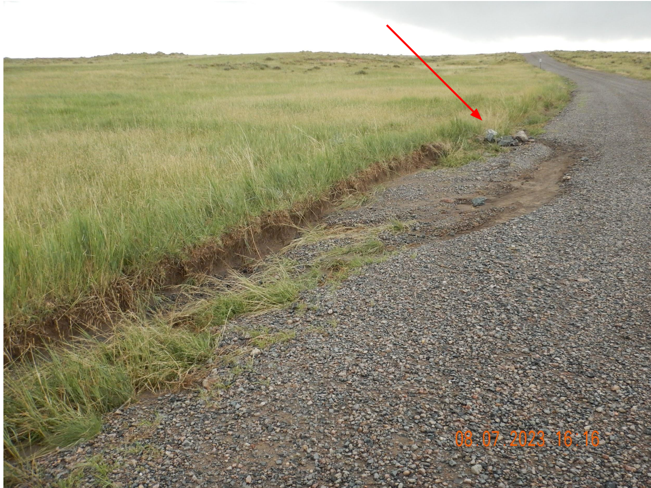
Photo 12. Photo illustrates another check dam BMP which is not in proper functioning condition and an example of increased erosion undercutting the bank of the lease road.
