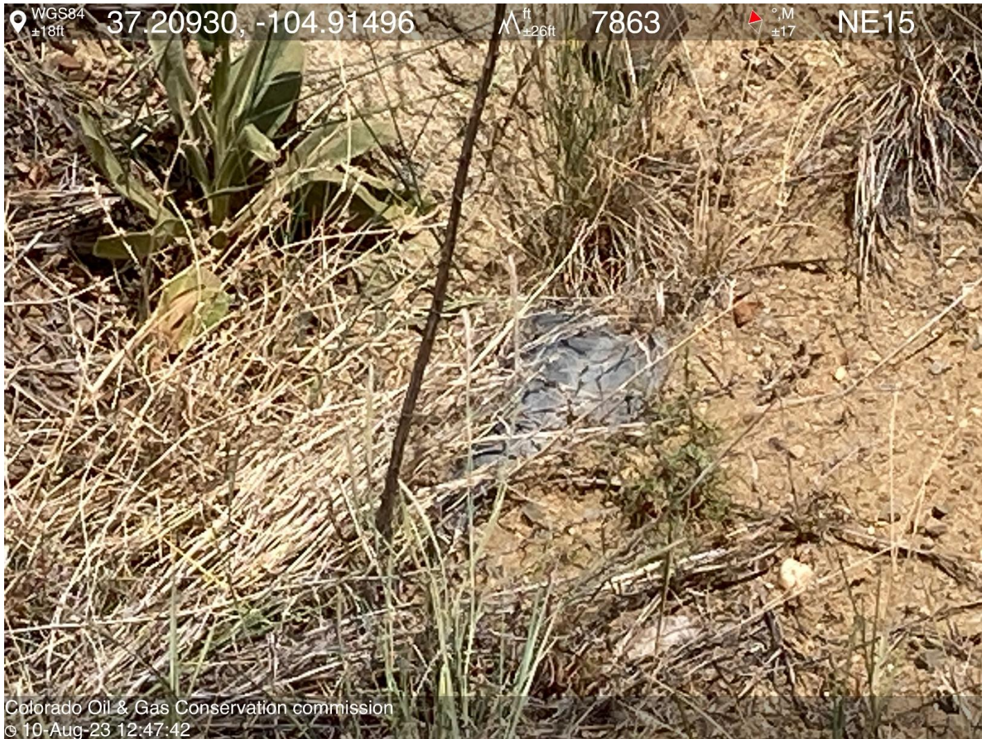
PHOTO 5: CULVERT APPROXIMATELY 200 YRD NORTH/ NORTHEAST OF LOCATION IS ALMOST COMPLETELY COVERED BY SEDIMENT. CLEAN AND MAINTAIN ALL CULVERTS ALONG ROW ACCORDING TO RULE 1002. CA DATE 9-10/2023.
