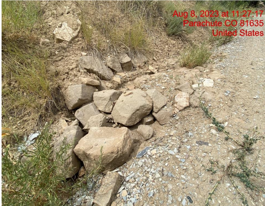
Check Dam Needs Maintenance – Photo #05692
