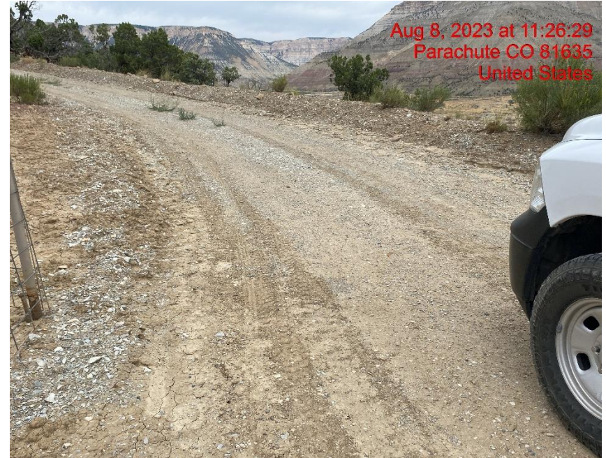
Insufficient Vehicle Tracking BMPs at Location Entrance/Exit – Photo #05691
