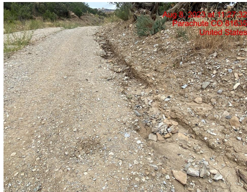
Rill Erosion Cutting Through Lease Road – Photo #05694
