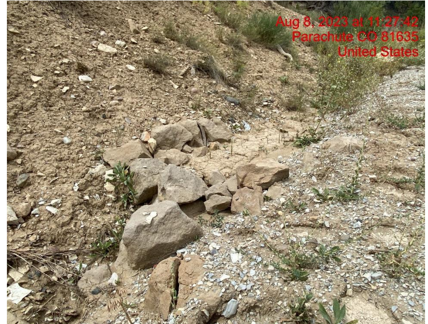
Check Dam Needs Maintenance – Photo #05695
