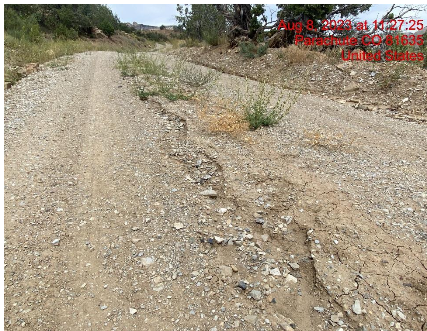
Rill Erosion Cutting Through Lease Road – Photo #05693
