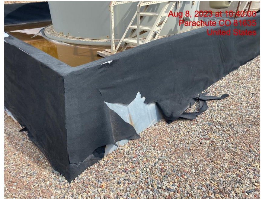
Damaged Berm Liner – Photo #05667
