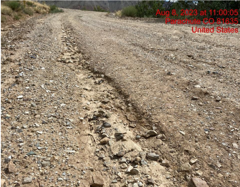
Rill Erosion Cutting Through Lease Road – Photo #05674
