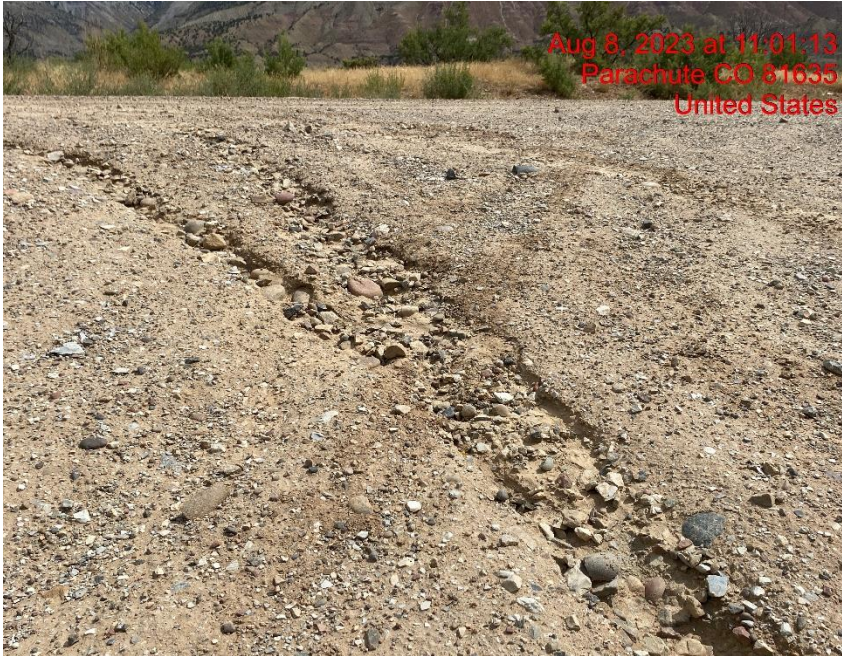
Rill Erosion Cutting Through Lease Road – Photo #05677
