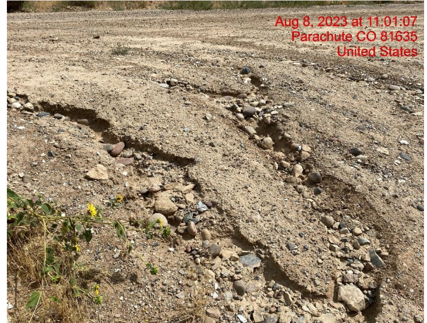
Rill Erosion Cutting Through Lease Road – Photo #05676
