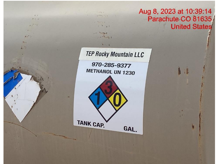
Methanol Tank Label Does Not State Tank Capacity – Photo #05665
