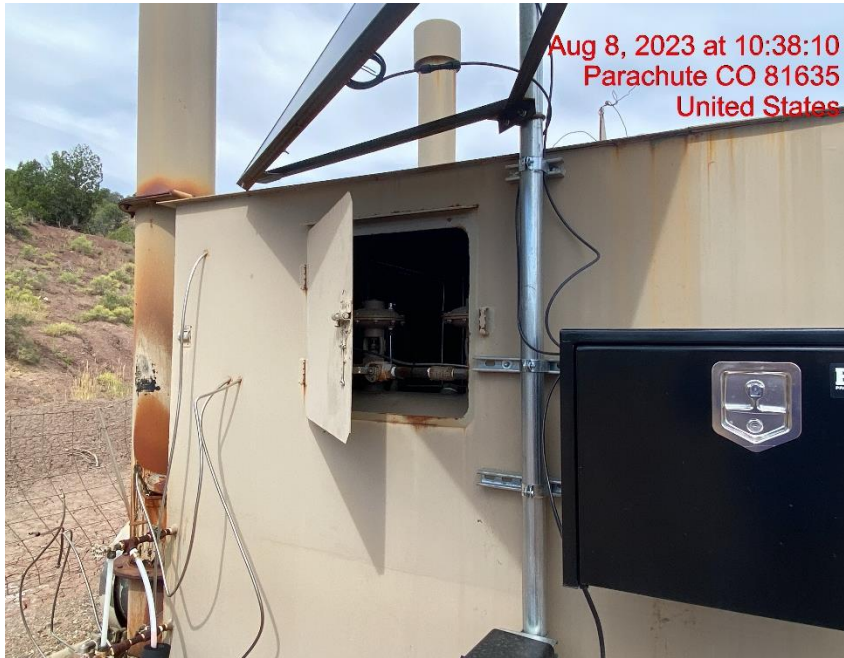
Separator Hatch Unsecured – Photo #05663
