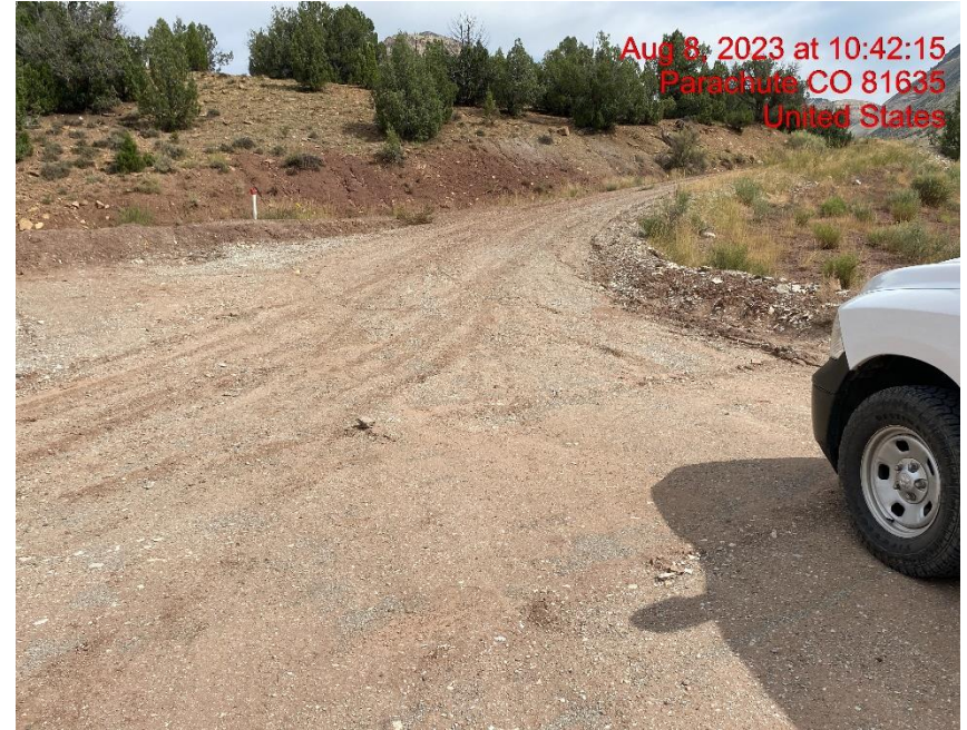
Insufficient Vehicle Tracking BMPs at Location Entrance/Exit – Photo #05672
