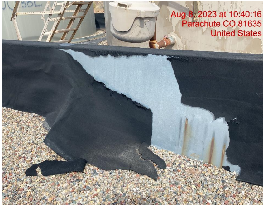
Damaged Berm Liner – Photo #05668
