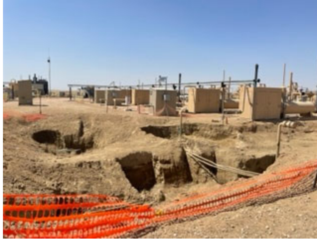
11 – Wells Ranch AE20 east, west and meter skid excavation extents
