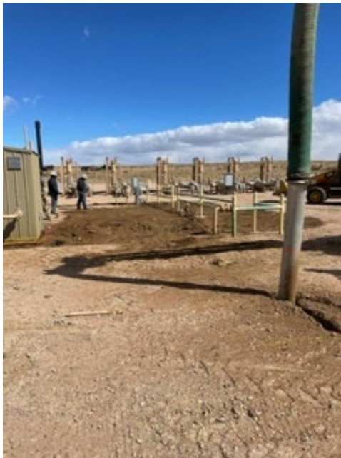
2 – Wells Ranch AE20 stained soil pot holing, south of the initial location where free product surfaced
