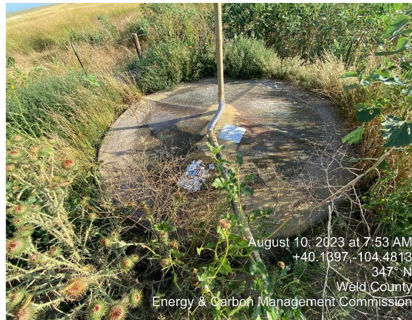
Weathered NFPA placard/ Missing capacity label
