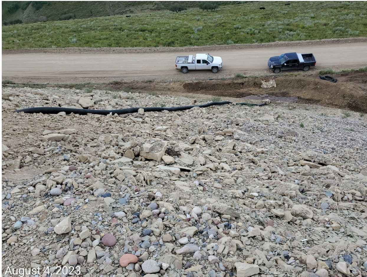
Photo 15: Photo example showing slope drain has not been properly secured per good engineering practices.
