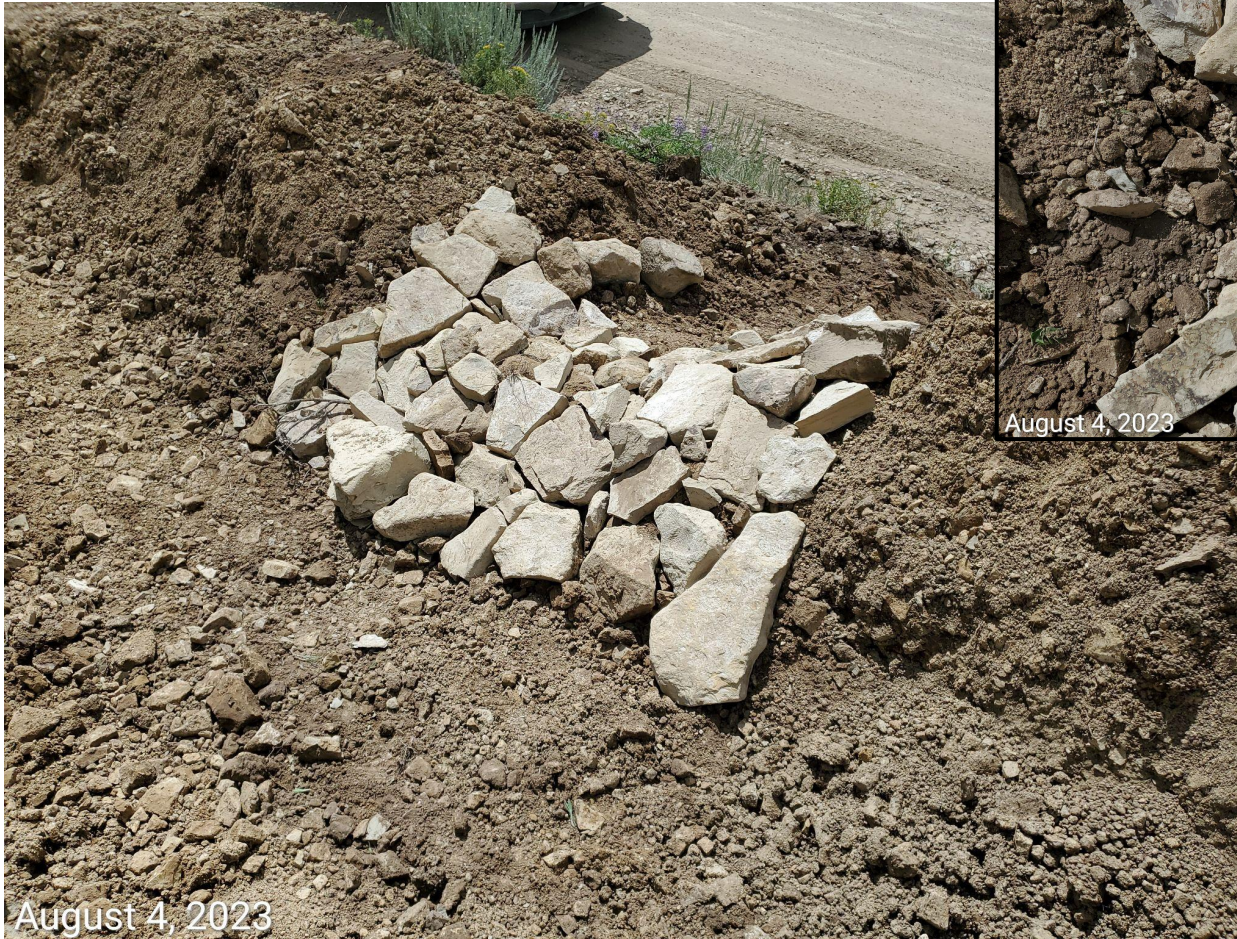
Photo 19: Photo shows outlet/spillway of the sediment trap. Control has been constructed per good engineering practices; outlet only partially armored and not in conjunction with geotextile lining.
