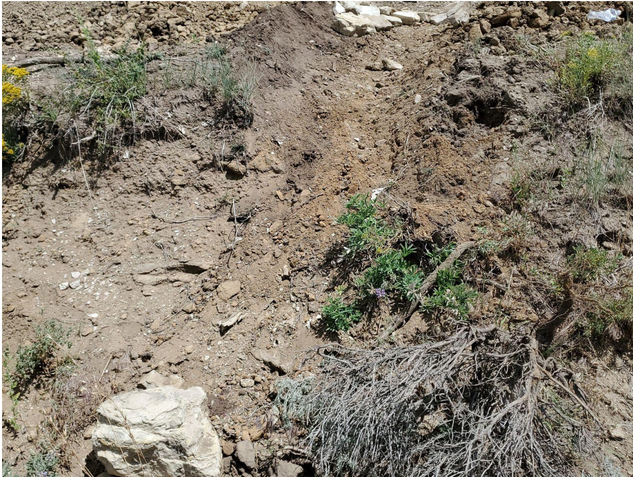
Photo 20: Photo shows outlet/spillway of the sediment trap. Control has been constructed per good engineering practices; outlet only partially armored and not in conjunction with geotextile lining.
