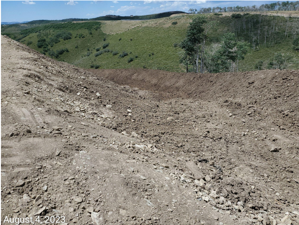
Photo 1: Photo taken from the north end of the Location, facing west. Photo shows Operator's attempts to remove the fill material from the topsoil stockpile. Photo also shows BMPs to ensure soils remain segregated, protected from weeds, wind and water erosion, as well as BMPs to stabilize, minimize degradation and sediment transport remain missing or insufficient.
