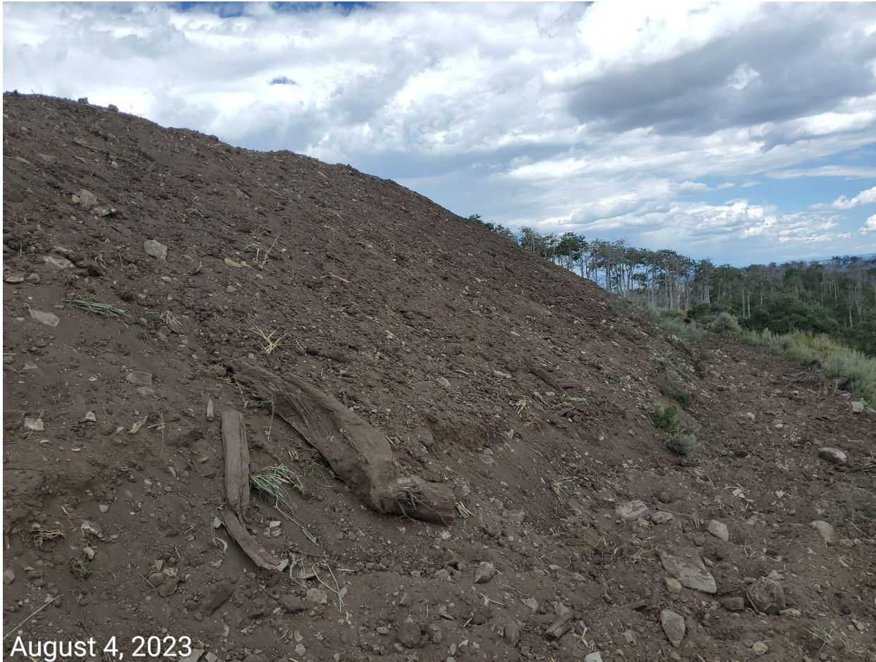
Photo 5: Photo shows BMPs to ensure soils remain segregated, protected from weeds, wind and water erosion, as well as BMPs to stabilize, minimize degradation and sediment transport remain missing or insufficient.
