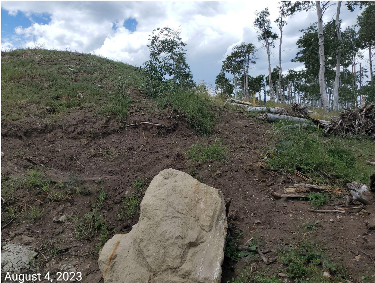
Photo 10: Photo taken from the east end of the Location. Photo shows BMPs to ensure soils remain segregated, protected from weeds, wind and water erosion, as well as BMPs to stabilize, minimize degradation and sediment transport remain missing or insufficient; Perimeter controls at stockpile (silt fence) completely removed.
