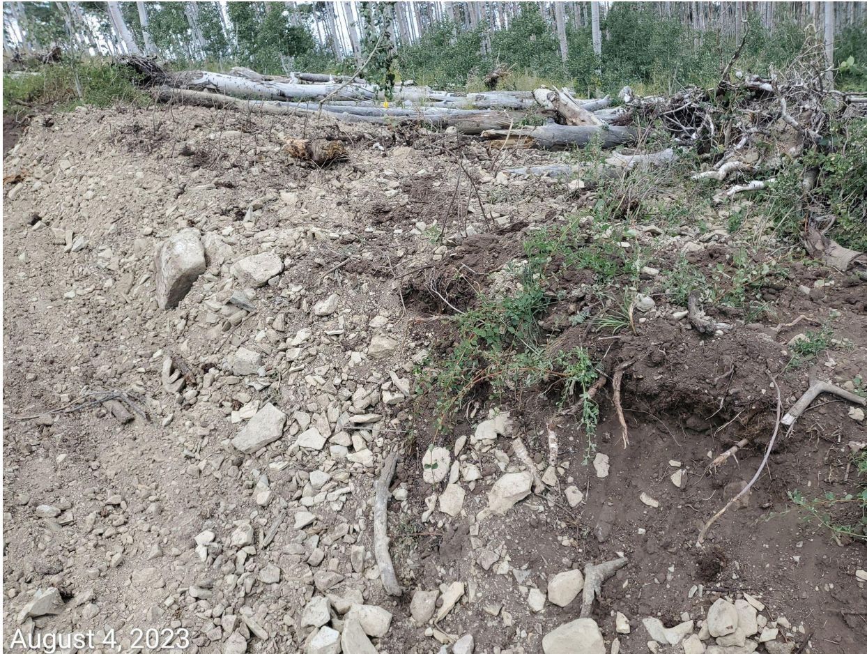
Photo 8: Fill material remains spread over topsoil and off-site.
