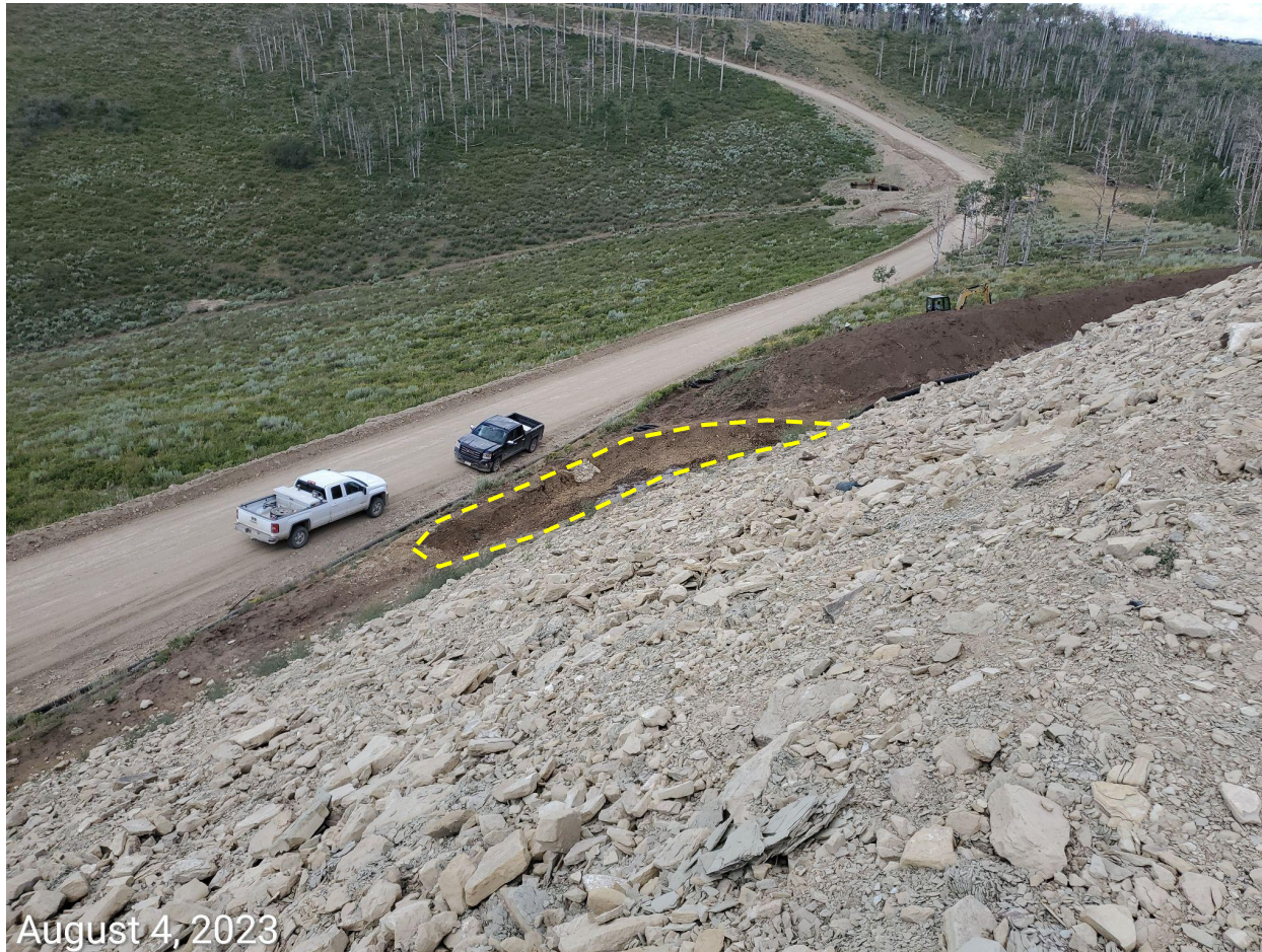
Photo 17: Photo taken from the west end of the Location. Photo shows a single sediment trap constructed on the west end of the location; control measure is inadequate in size to manage runoff from the 3.7 acre working pad.
