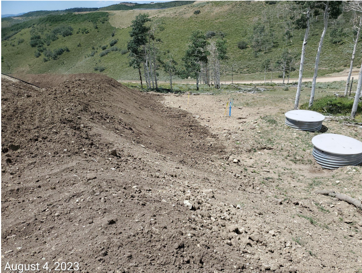
Photo 3: Photo of topsoil stockpile on the north end of the Location. Photo shows BMPs to ensure soils remain segregated, protected from weeds, wind and water erosion, as well as BMPs to stabilize, minimize degradation and sediment transport remain missing or insufficient.
