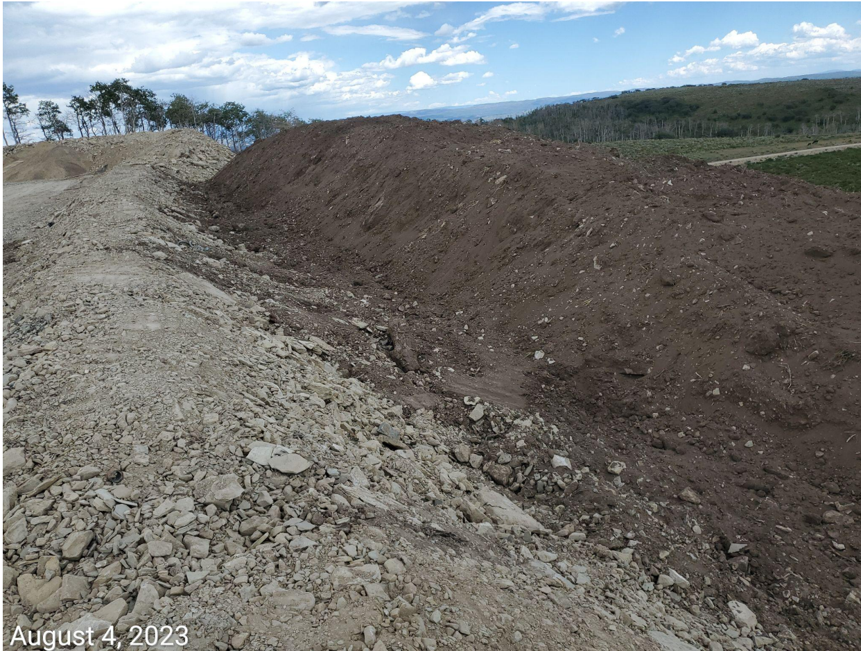
Photo 4: Photo taken from the south end of the Location, facing west. Photo shows Operator's attempts to remove the fill material from the topsoil stockpile. Photo also shows BMPs to ensure soils remain segregated, protected from weeds, wind and water erosion, as well as BMPs to stabilize, minimize degradation and sediment transport remain missing or insufficient.
