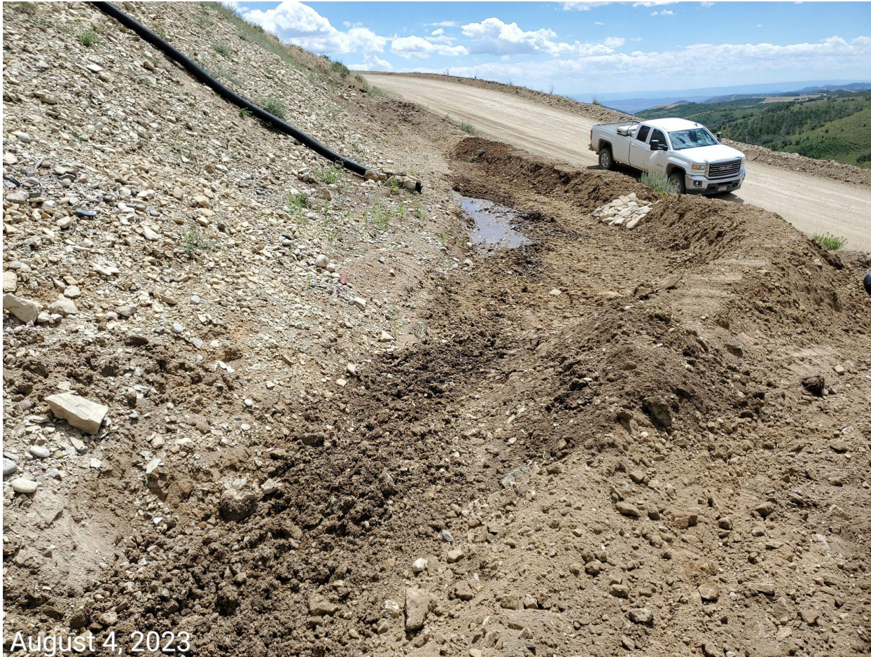
Photo 18: Photo taken from the sediment trap on the west end of the Location. Control measure is inadequate in size to manage runoff from the 3.7 acre working pad.
