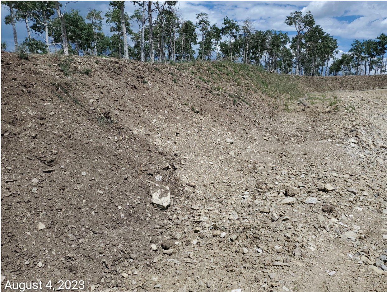
Photo 2: Photo of topsoil stockpile on the north end of the Location. Photo shows BMPs to ensure soils remain segregated, protected from weeds, wind and water erosion, as well as BMPs to stabilize, minimize degradation and sediment transport remain missing or insufficient.
