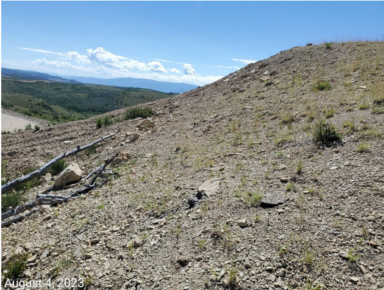
Photo 15: Photo taken from the interim areas on the north end of the Location, facing southeast. Photo shows bare and unstabilized soils; perimeter control measures to manage runoff not observed; interim areas not progressing towards 1003 standards.
