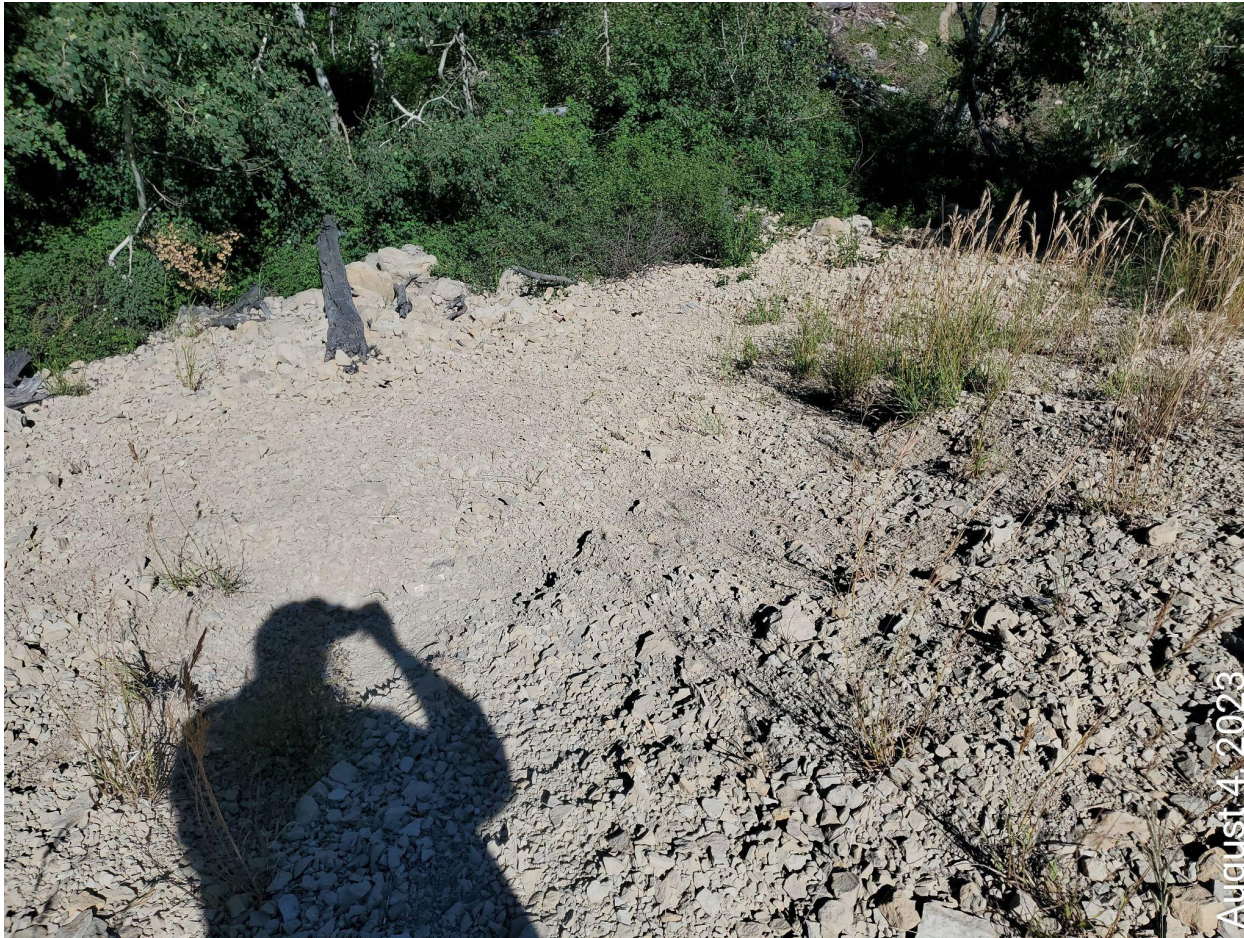
Photo 14: Photo shows bare and unstabilized soils; perimeter control measures to manage runoff not observed; interim areas not progressing towards 1003 standards. Sediment/fill material encroachment onto vegetation within adjacent areas of the Location.
