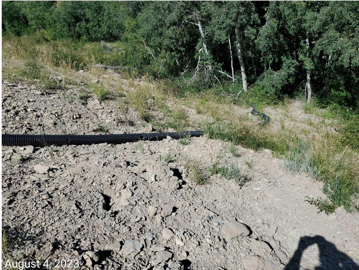
Photo 9: Slope drain has not been secured in accordance with good engineering practices.
