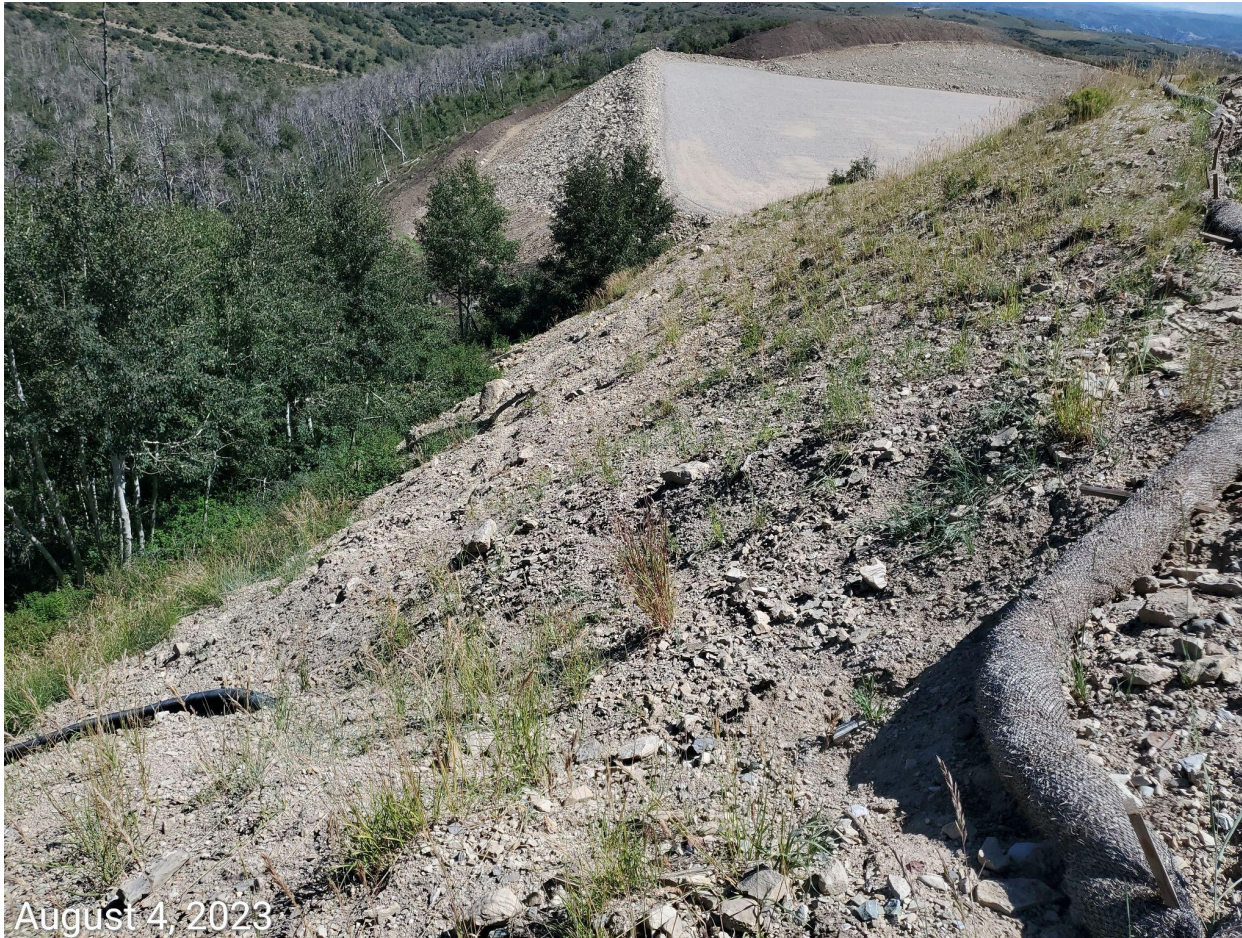
Photo 7: Photo taken from the interim areas on the northwest end of the Location, facing northeast. Interim areas are not progressing towards an 80% uniform desirable perennial vegetative cover to that of the adjacent reference.
