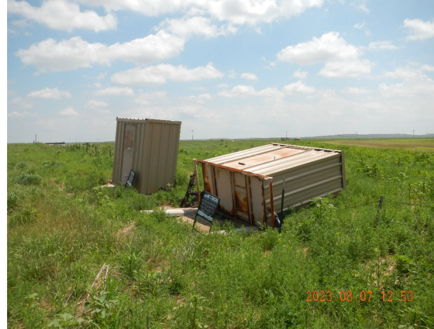
10. View of remote Meter Run location with Meter House for the Schneller 10-22-5-45 already blown over. Note vegetation.
