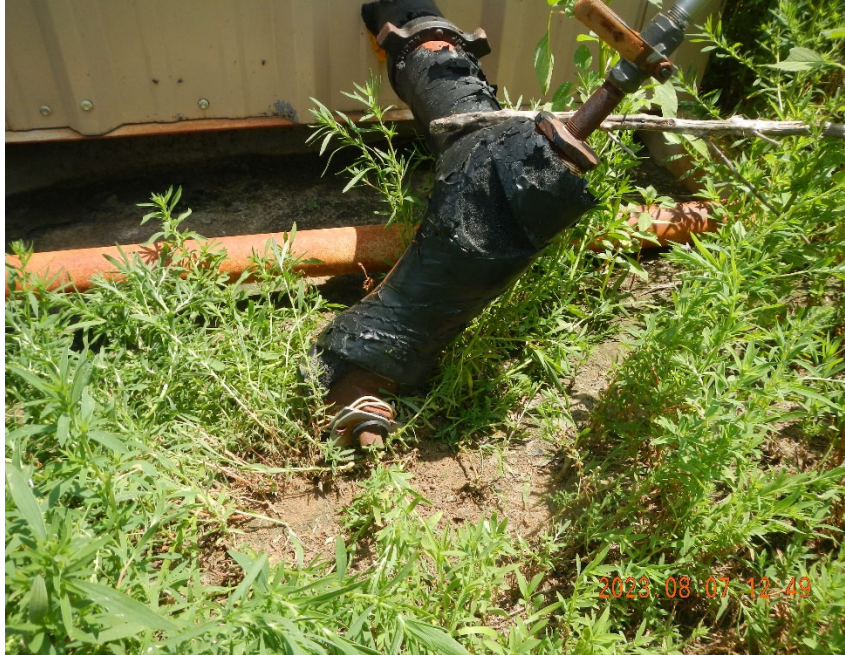
7. Inlet flowline being bent due to Meter Shed leaning. Note vegetation.
