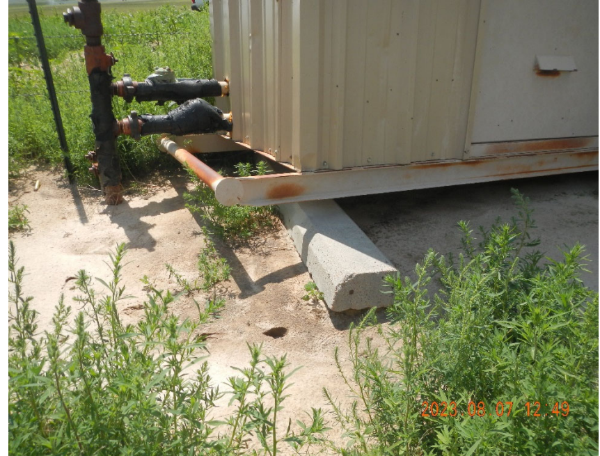
6. Meter Shed coming off supports and leaning backwards placing tension on the flowlines.
