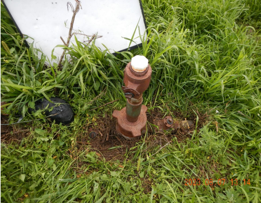
3. View of Wellhead and Casing valves.
