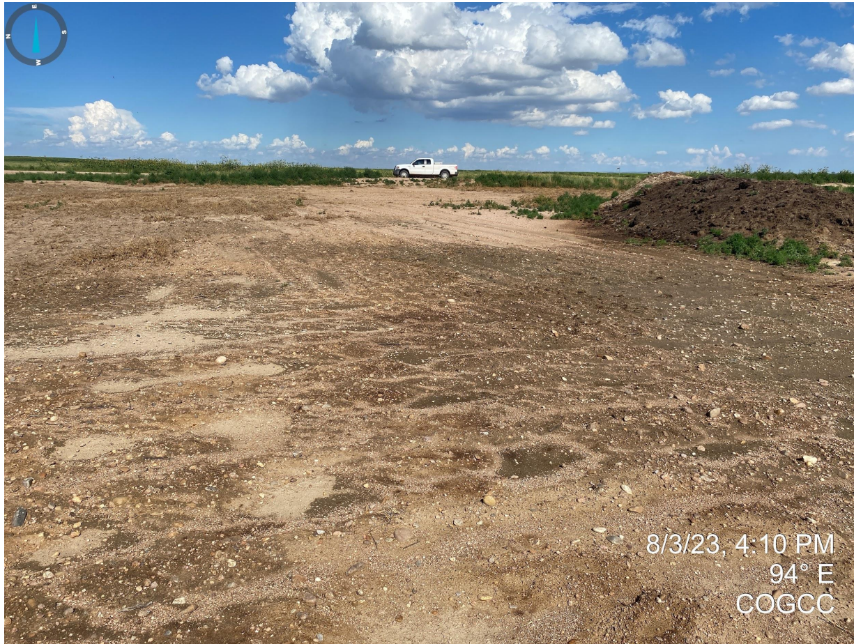
Photo 2. Continued from Photo 1. Road base and gravel remain on the location and requires removal per Rule 1004.
