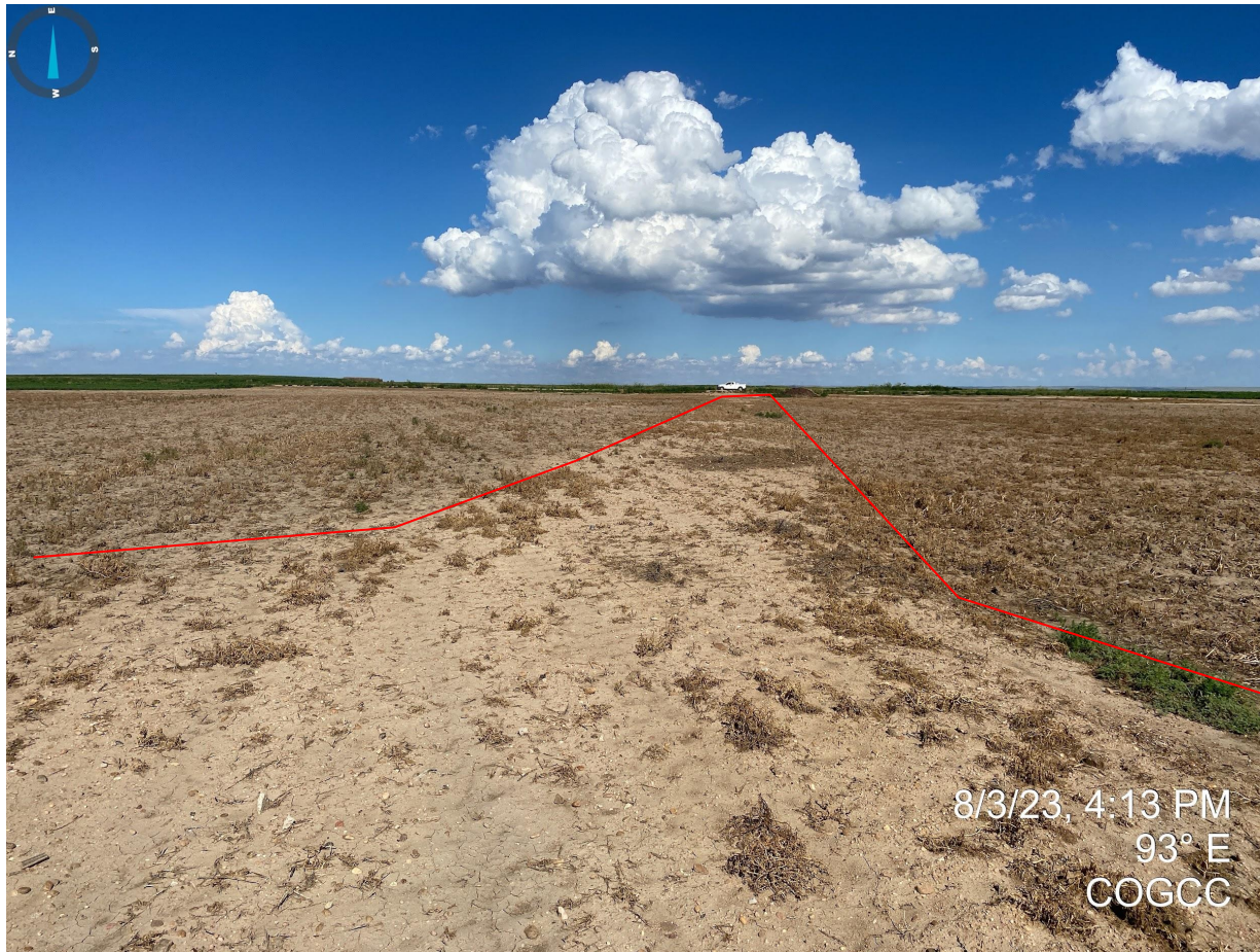
Photo 7. Taken from the former well head. Red outline illustrates the access road that requires additional reclamation activities including but not limited to- recontouring/grading, leveling, removal of road base/gravel, and decompaction.
