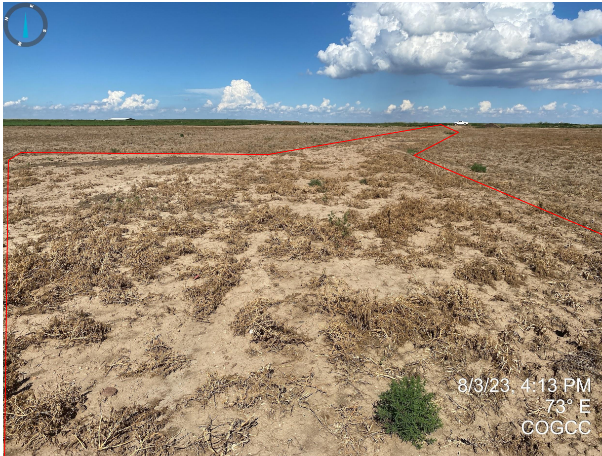
Photo 8. Taken from the former well location. The former well location will requires additional reclamation activities including but not limited to- recontouring/grading, leveling, removal of road base/gravel, and decompaction.
