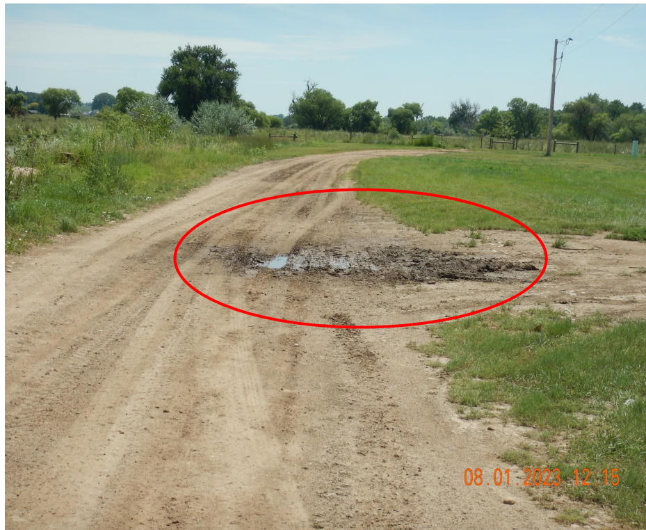
Photo 4. Photo taken from a portion of the access road, facing East. Photo illustrates road damages from plugging operations.
