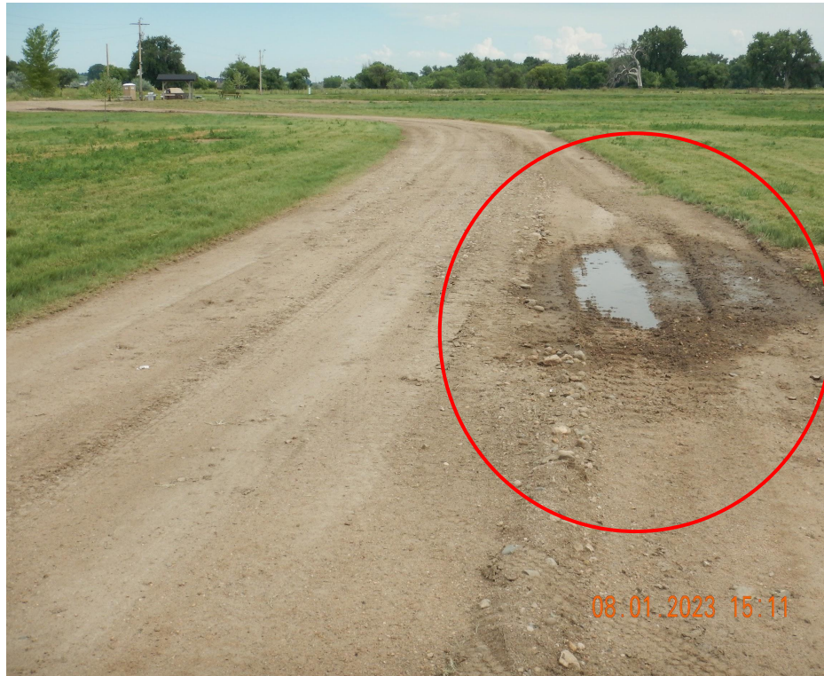
Photo 2. Photo taken from a portion of the access road, facing Southeast. Photo illustrates road damages from plugging operations.
