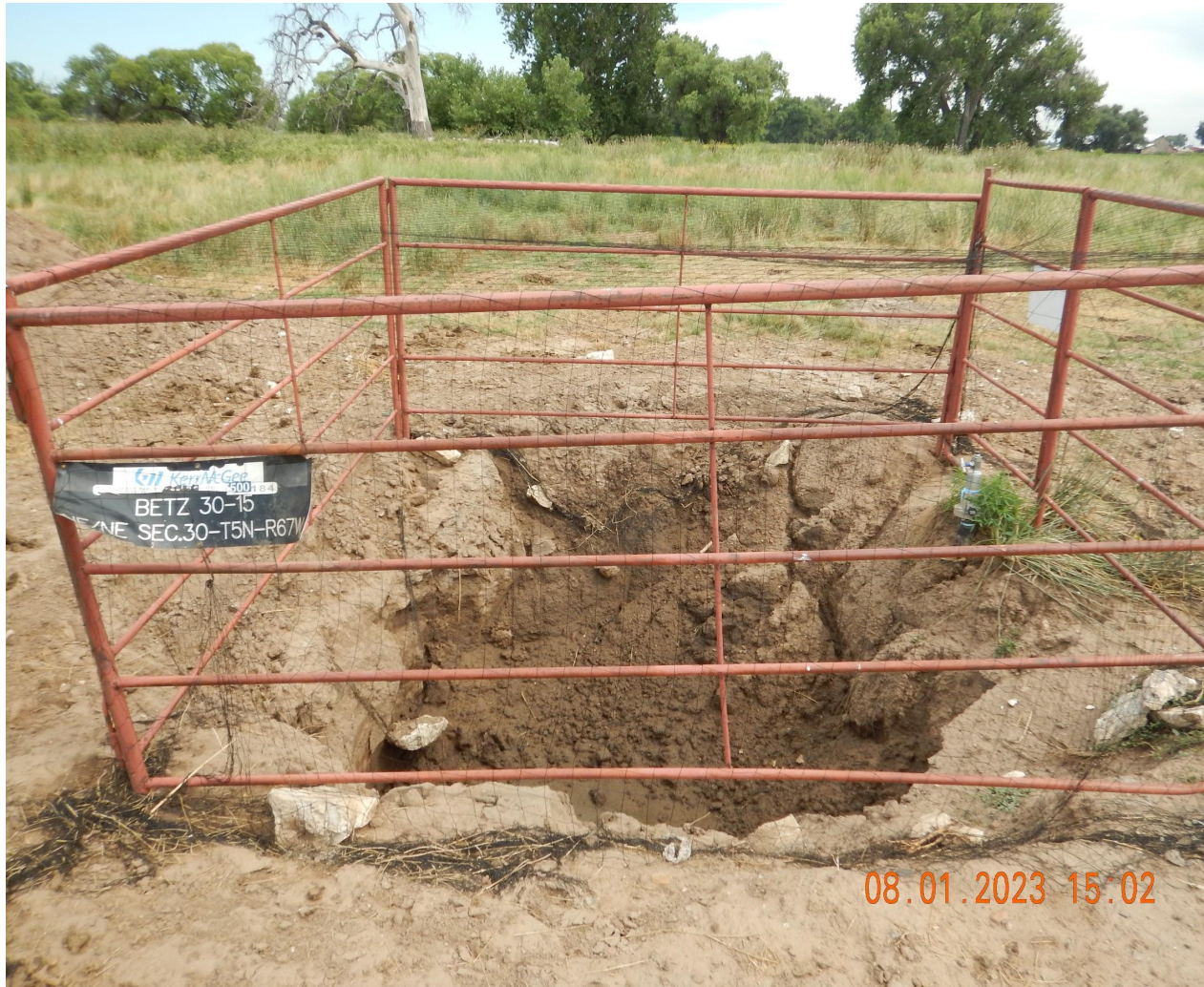
Photo 6. Photo taken from the well location, facing East. Photo illustrates an open excavation due to plugging operations. Cattle fencing and netting have been installed. Netting is in need of repair as approximate 10" holes were observed.
