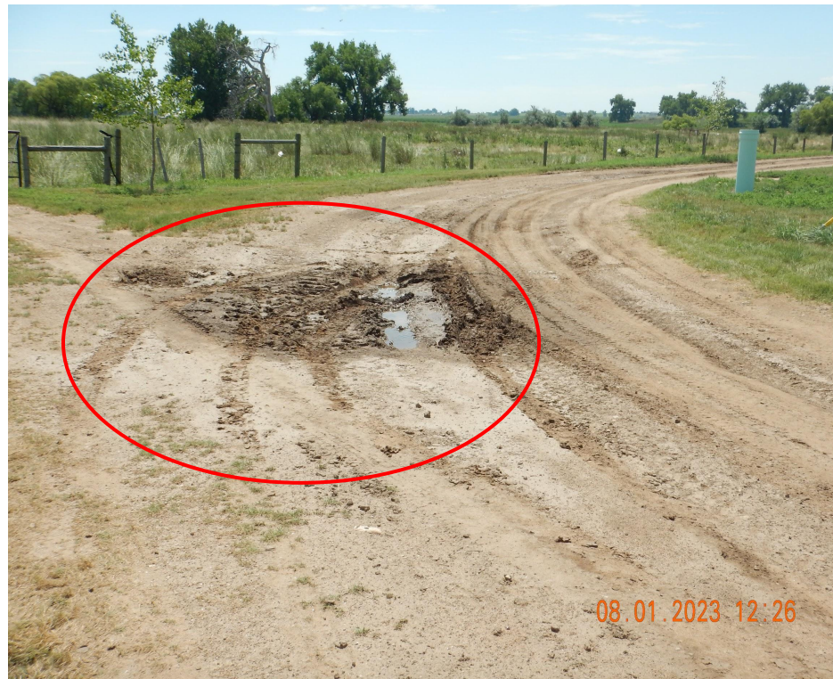
Photo 5. Photo taken from a portion of the access road, facing East. Photo illustrates road damages from plugging operations.
