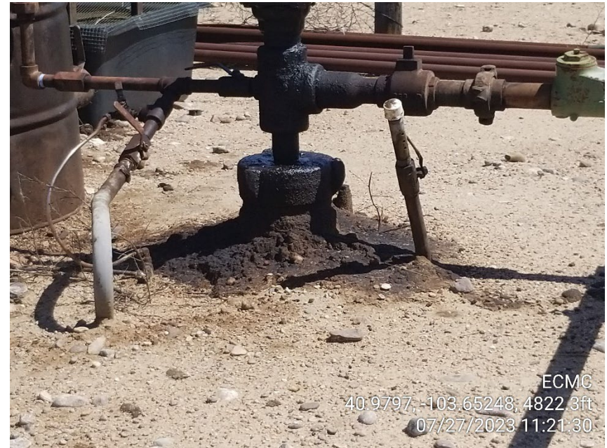
Photo 2 – Wellhead – Stained Soil
