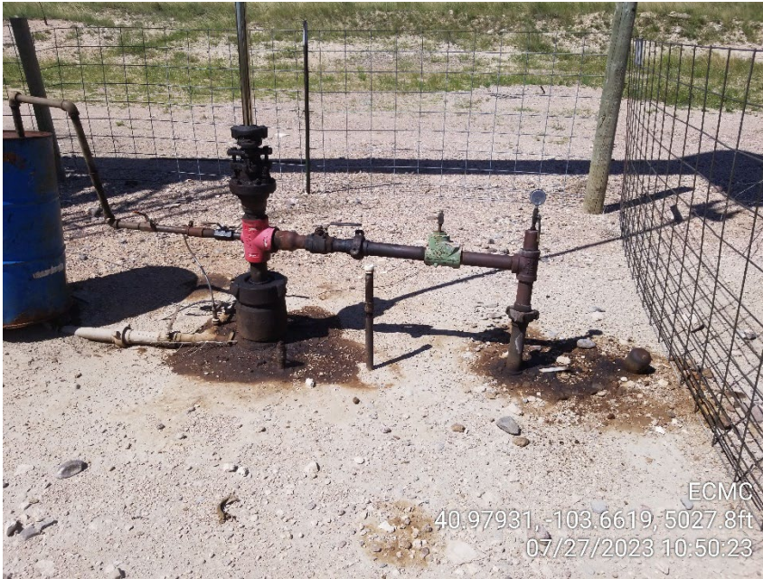
Photo 3 – Wellhead – Stained Soil
