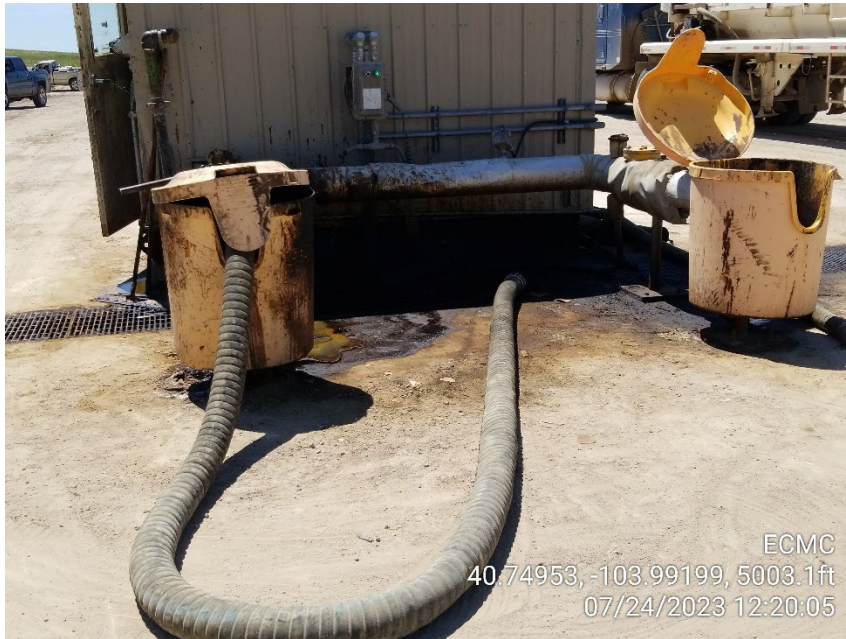
Photo 13 – Stained Soil and Oily Waste at Truck Load Outs
