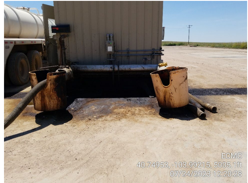
Photo 14 – Stained Soil and Oily Waste at Truck Load Outs
