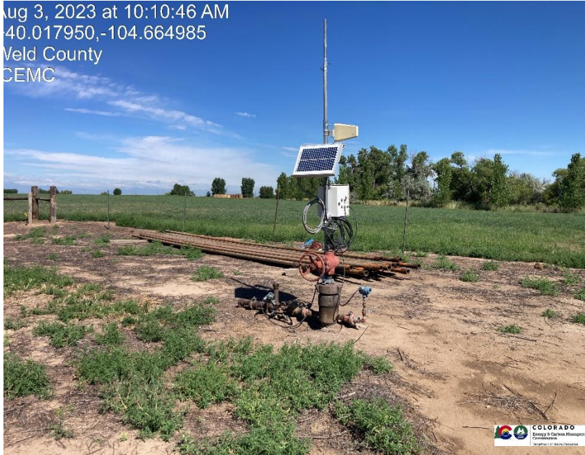
Pic 1 wellhead sign missing on wellhead / tubing on ground from offset mitigation
