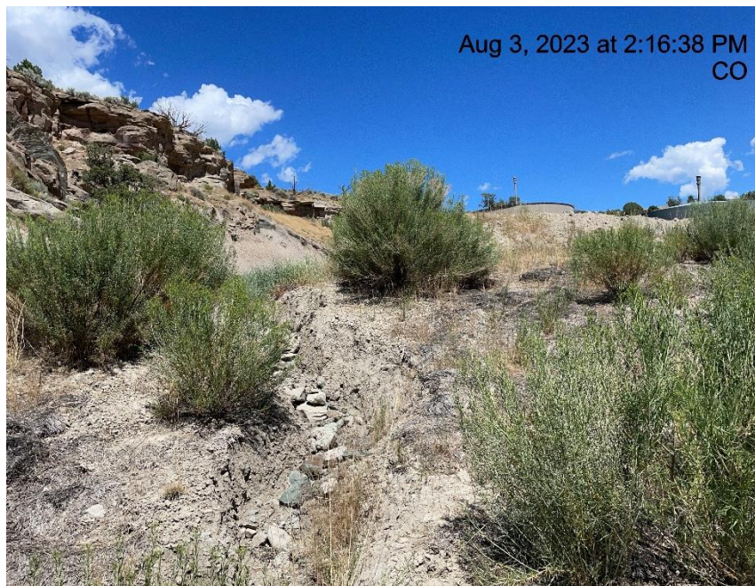
Photo # 4515 Erosion & transport of sediment/BMP's need maintenance (N/NW area of location on slope behind tank battery)
