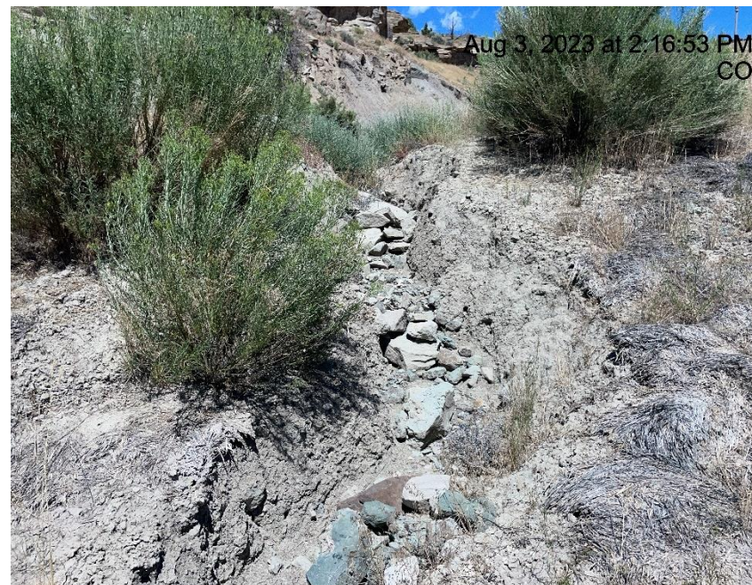
Photo # 4516 Erosion & transport of sediment/BMP's need maintenance (N/NW area of location on slope behind tank battery)
