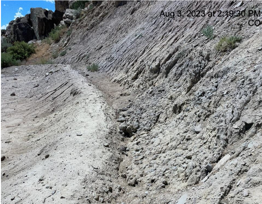
Photo # 4521 Ditch needs maintenance (N/NW area of location running along cut slope behind production separators)
