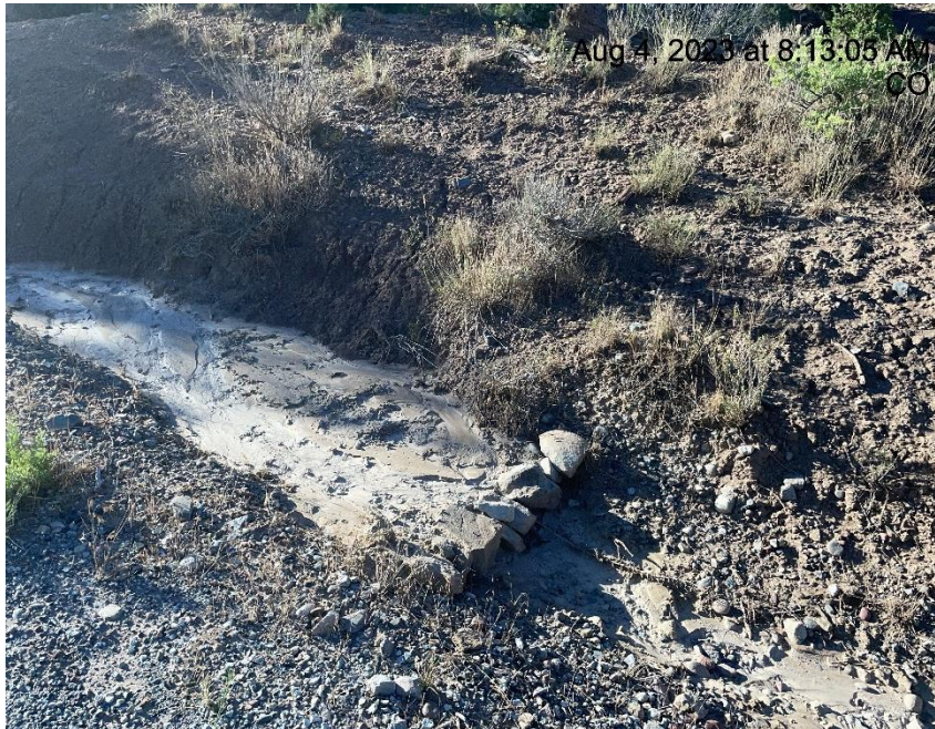
Photo # 4546 Check dam needs maintenance (S/SE area of location & road)
