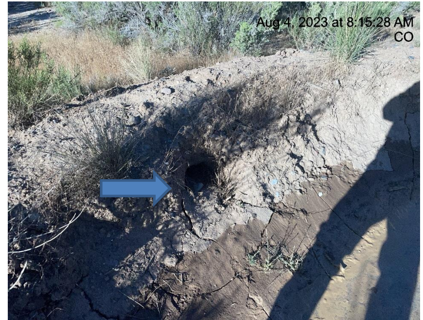
Photo # 4549 Sediment trap needs maintenance/tunnel erosion (S/SW area of location down from the check dams)
