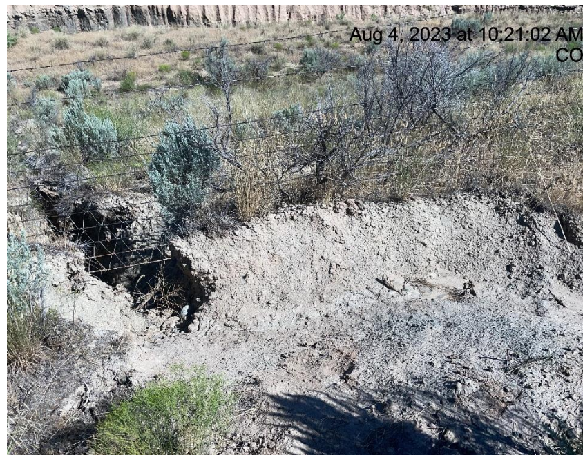
Photo # 4683 Insufficient run off controls/BMP's/erosion & transport of sediment
