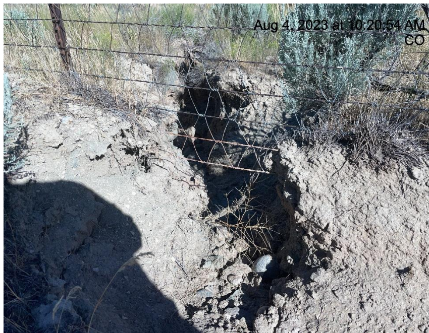
Photo # 4681 Insufficient run off controls/BMP's/erosion & transport of sediment
