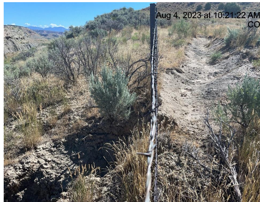
Photo # 4685 Insufficient run off controls/BMP's/erosion & transport of sediment
