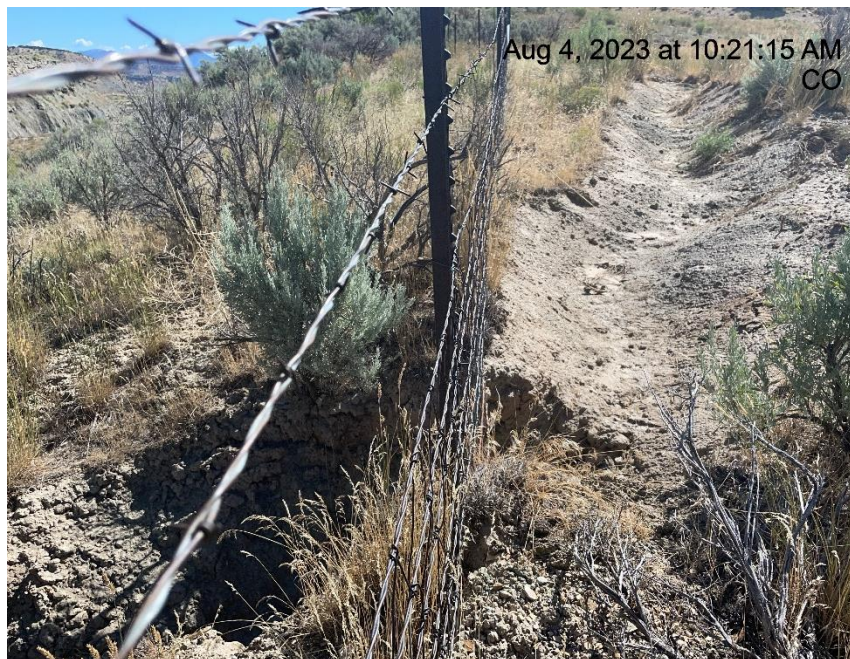
Photo # 4684 Insufficient run off controls/BMP's/erosion & transport of sediment
