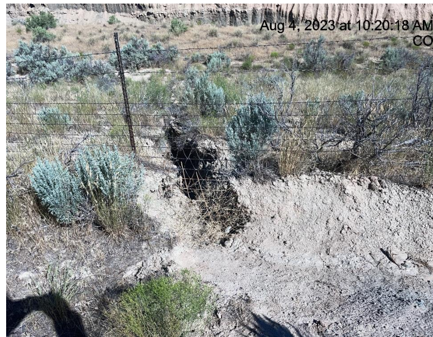
Photo # 4680 Ditch coming out sediment trap/insufficient run off controls/BMP's/erosion & transport of sediment
