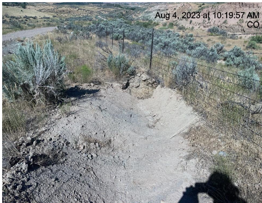
Photo # 4677 Insufficient run off controls/BMP's
