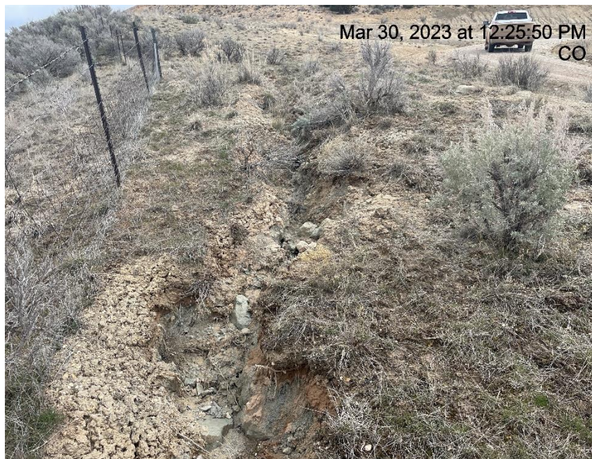
Photo # 3790 From inspection 708900206 conducted on 03/30/2023 Ditch coming out sediment trap/insufficient run off controls/BMP's/erosion & transport of sediment
