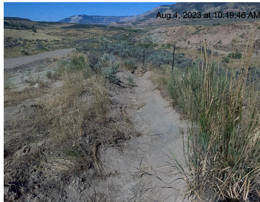
Photo # 4676 Ditch coming out sediment trap/insufficient run off controls/BMP's
