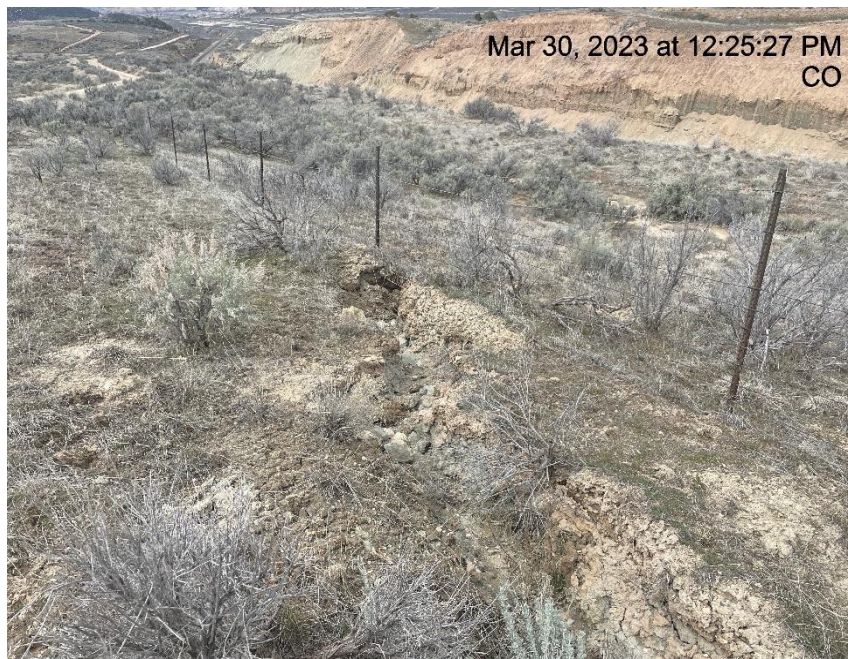
Photo # 3788 From inspection 708900206 conducted on 03/30/2023 Ditch coming out sediment trap/insufficient run off controls/BMP's/erosion & transport of sediment
