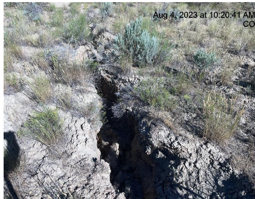
Photo # 4682 Insufficient run off controls/BMP's/erosion & transport of sediment
