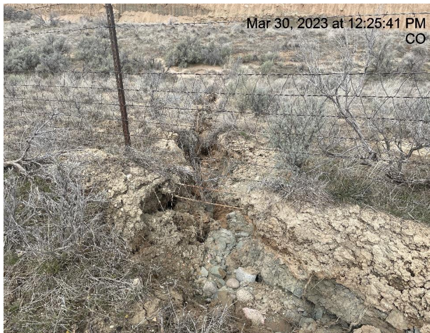
Photo # 3789 From inspection 708900206 conducted on 03/30/2023 Ditch coming out sediment trap/insufficient run off controls/BMP's/erosion & transport of sediment
