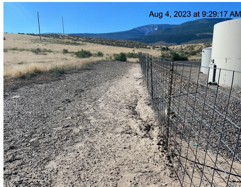
Photo # 4610 Erosion & transport of sediment
