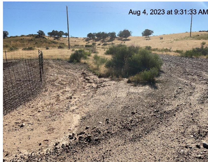
Photo # 4612 Erosion & transport of sediment off location onto lease road/insufficient run on/run off controls/BMP's
