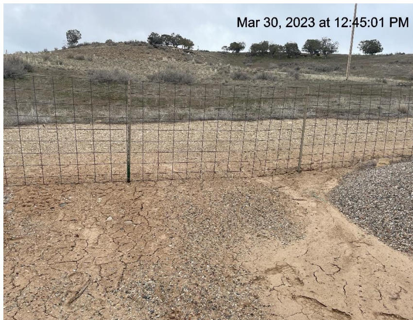
Photo #3814 From inspection 708900191 conducted on 03/30/2023 Erosion & transport of sediment
