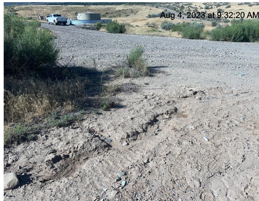
Photo # 4617 Erosion & transport of sediment off location onto lease road/insufficient run on/run off controls/BMP's
