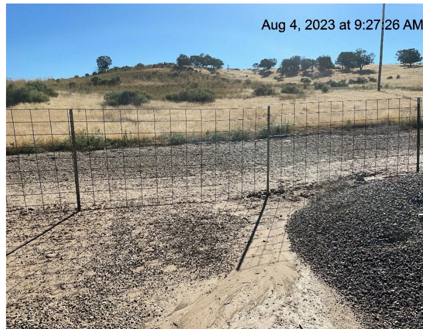
Photo # 4606 Erosion & transport of sediment
