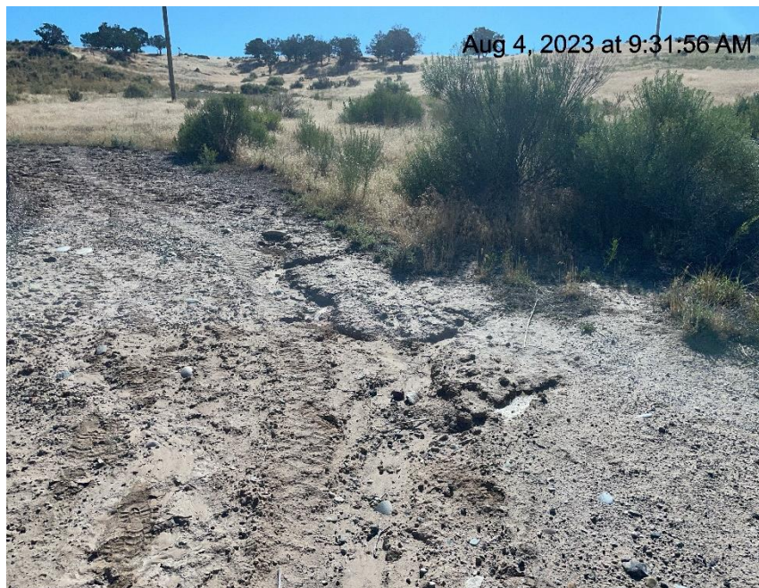
Photo # 4615 Erosion & transport of sediment off location onto lease road/insufficient run on/run off controls/BMP's
