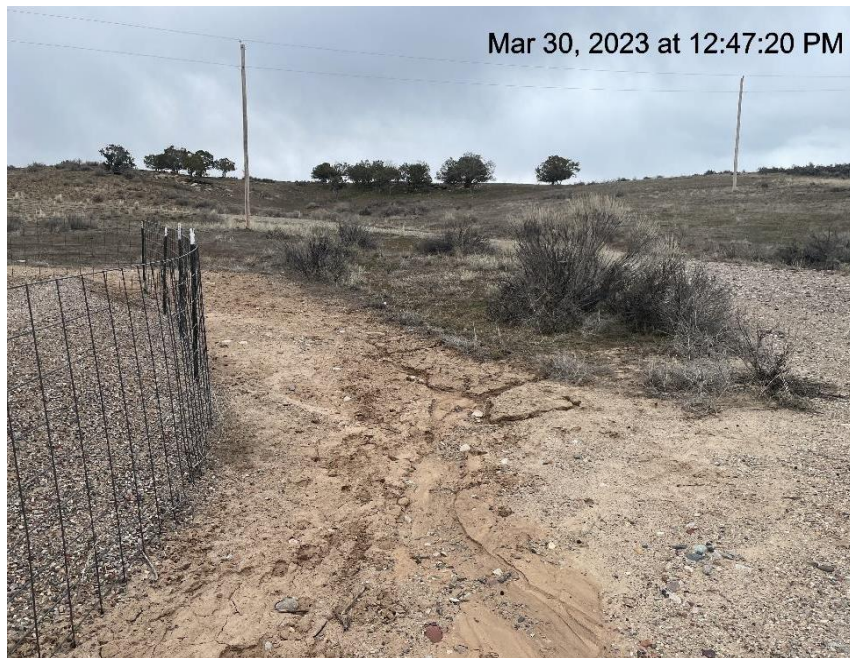
Photo # 3820 From inspection 708900191 conducted on 03/30/2023 Erosion & transport of sediment off location onto lease road/insufficient run on/run off controls/BMP's
