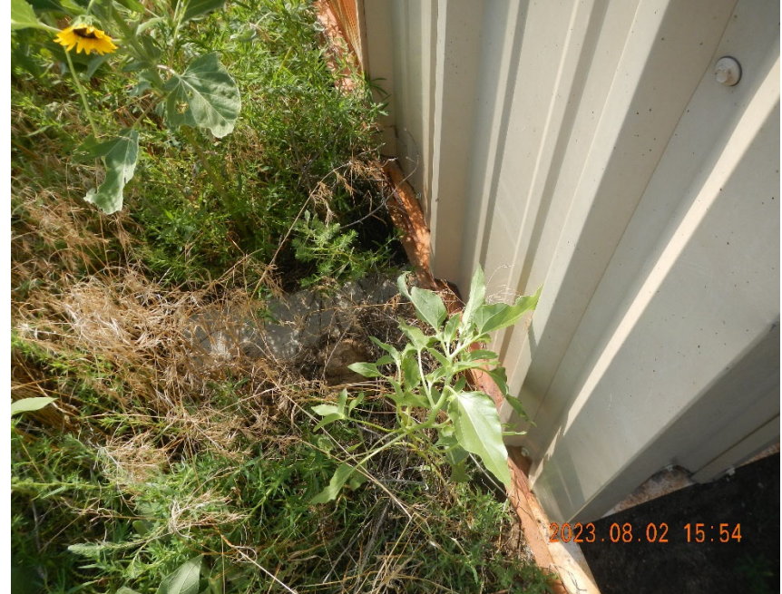
8. View of partially visible support piling. Meter has been blown partially off support and leaning. Note vegetation.
