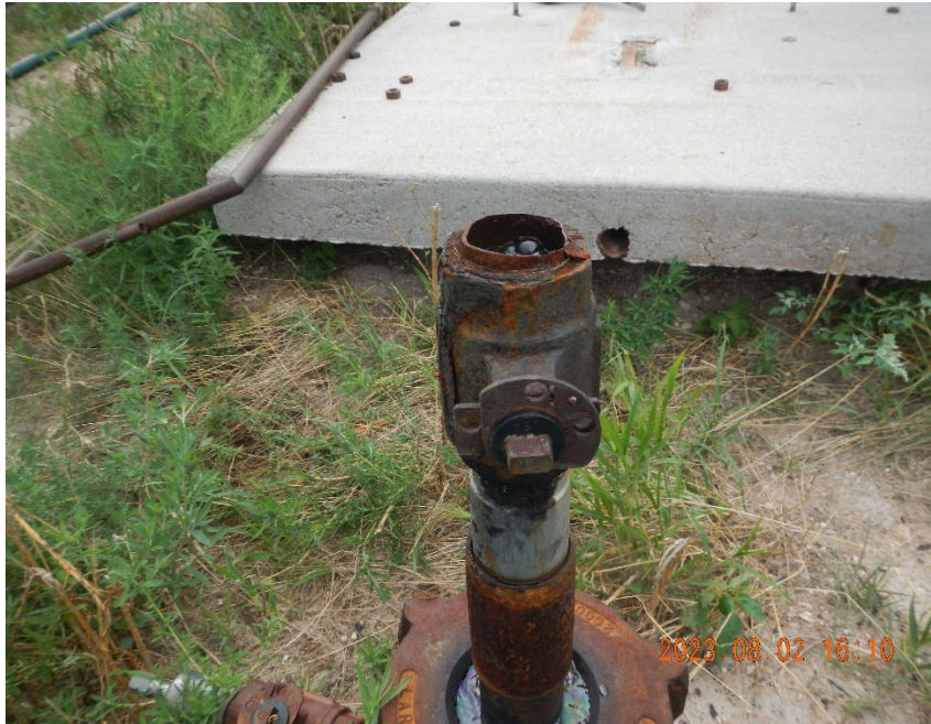
3. Unplugged open ended valve on end of tubing joint that is leaking. Bubble is visible in trapped water.
