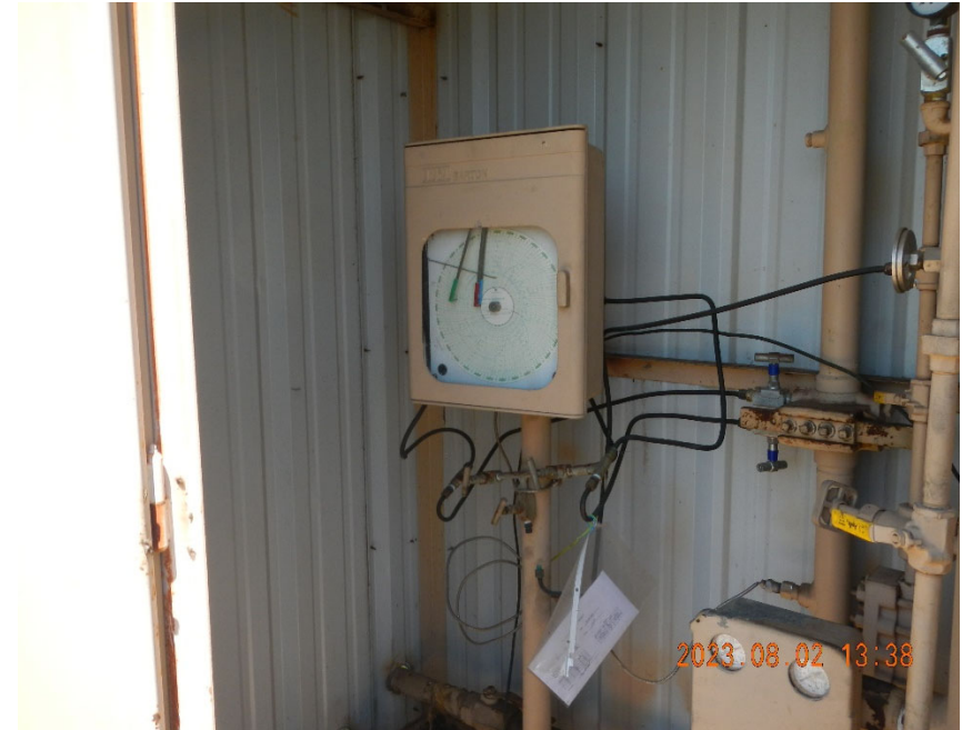
6. Gas Meter located inside Meter Shed.
