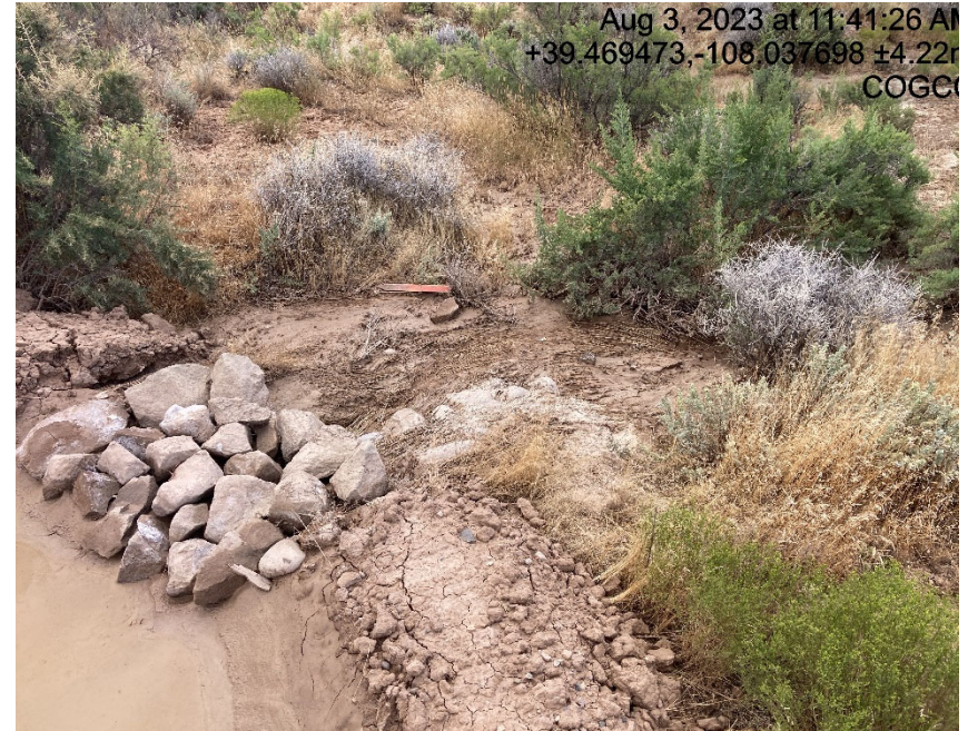
Sediment trap with sediment running over
