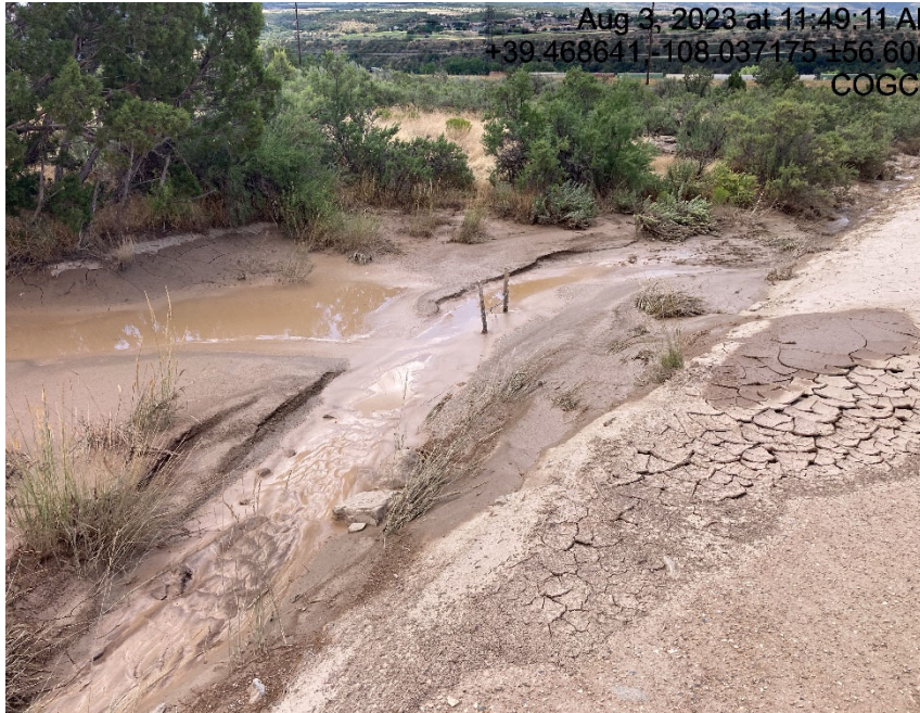
Inlet of culvert under sediment
