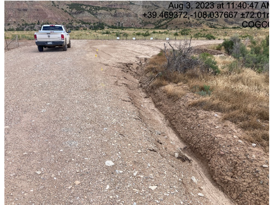
Gully erosion in ditch
