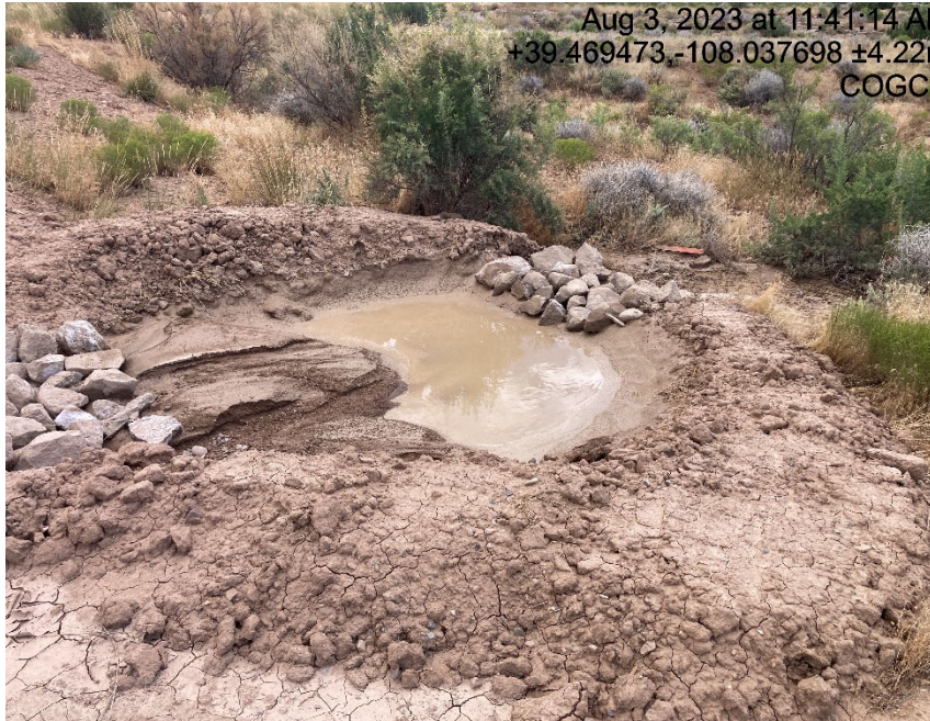
Sediment trap with sediment running over
