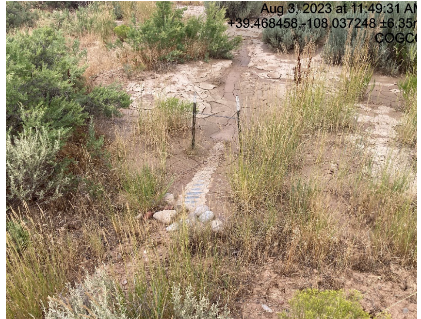
Outlet of culvert under sediment
