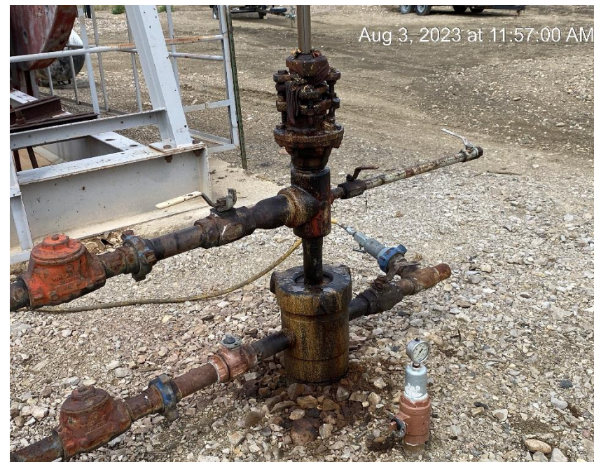
Wellhead leaks. Stained soil
