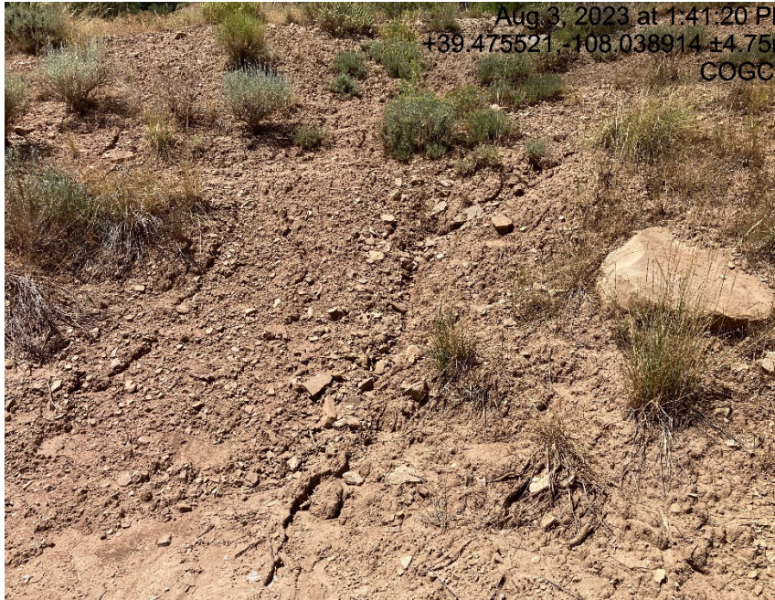
Cut slope erosion
