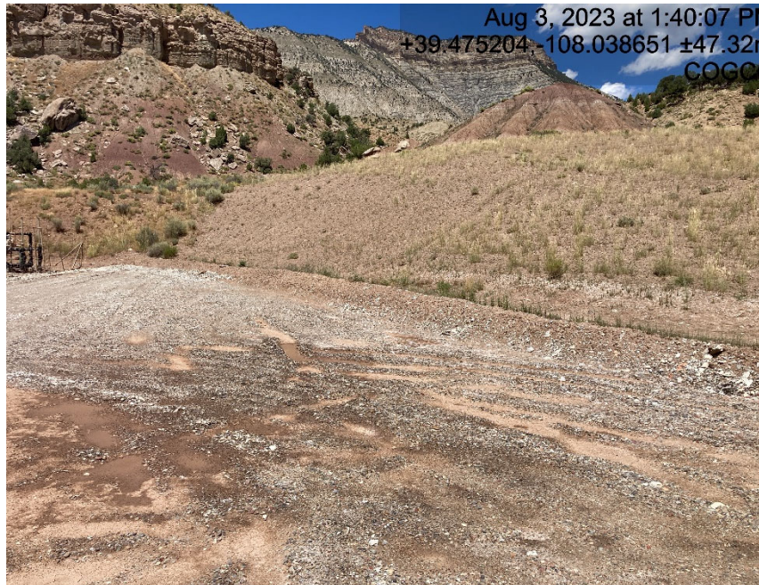
Cut slope erosion
