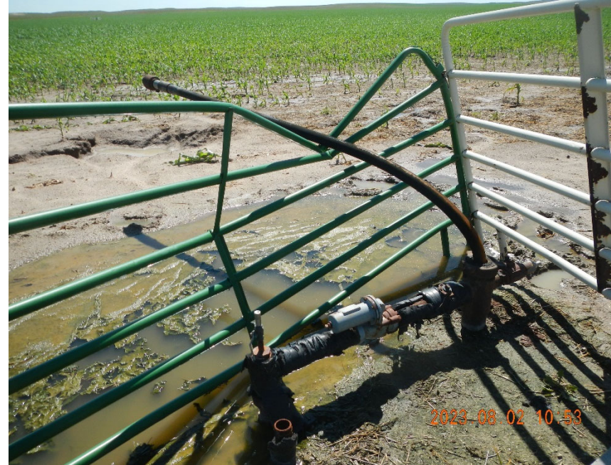
4. Closer view of bent tubing joint.
