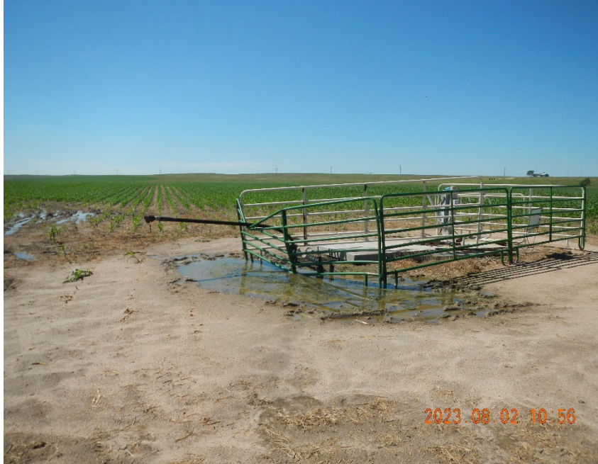
3. View of well location with tubing joint bent over.
