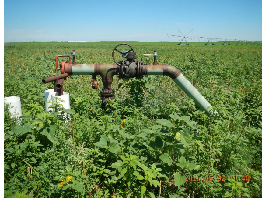
10. Pig Station on N side of Meter Shed. Note vegetation growth.
