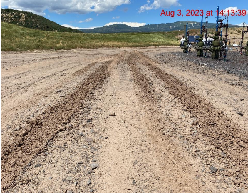
Location Lacks Stabilization – Photo #05474
