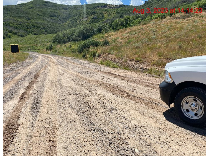
Insufficient Vehicle Tracking BMPs at Location Entrance/Exit – Photo #05475
