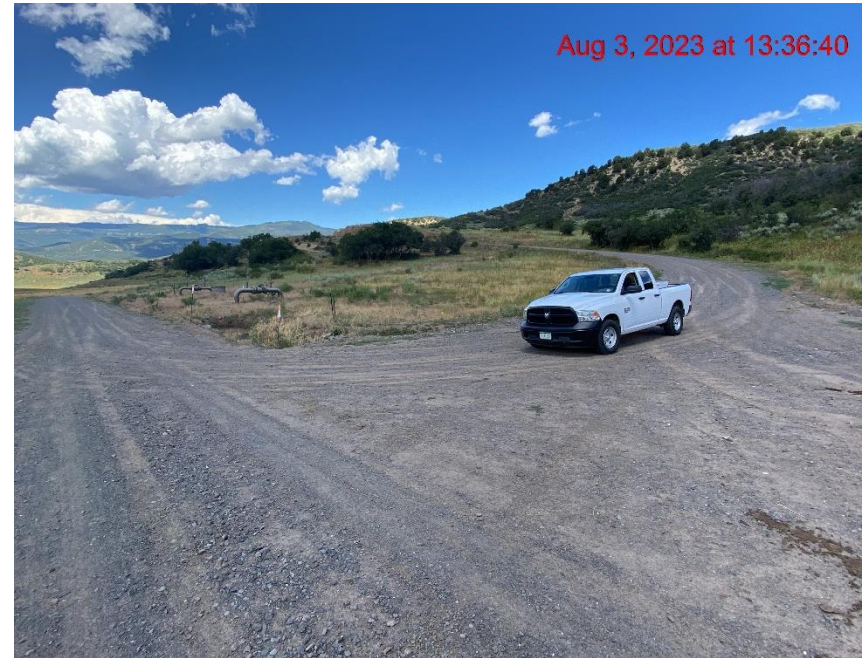
Insufficient Vehicle Tracking BMPs at Access Road Entrance/Exit – Photo #05445
