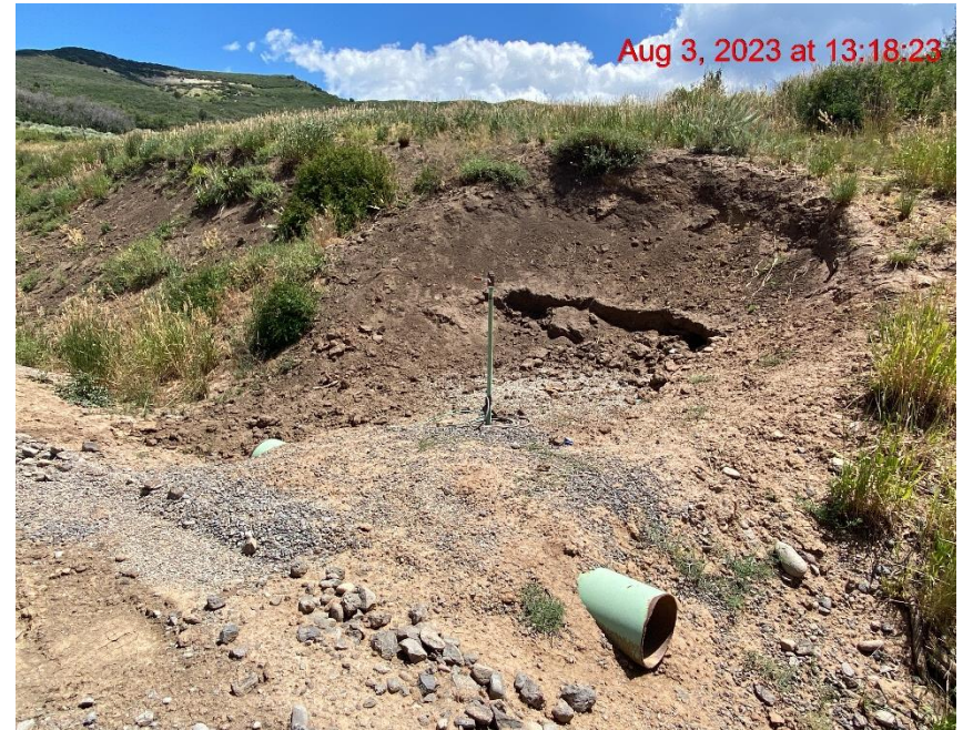
Insufficient Cut Slope Erosion Control – Photo #05442
