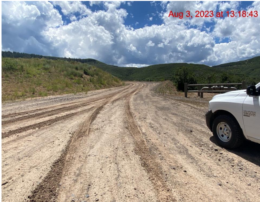
Insufficient Vehicle Tracking BMPs at Location Entrance/Exit – Photo #05443
