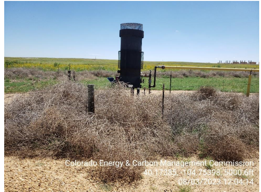
Photo 6 Tumble weeds accumulated around the ECD.
