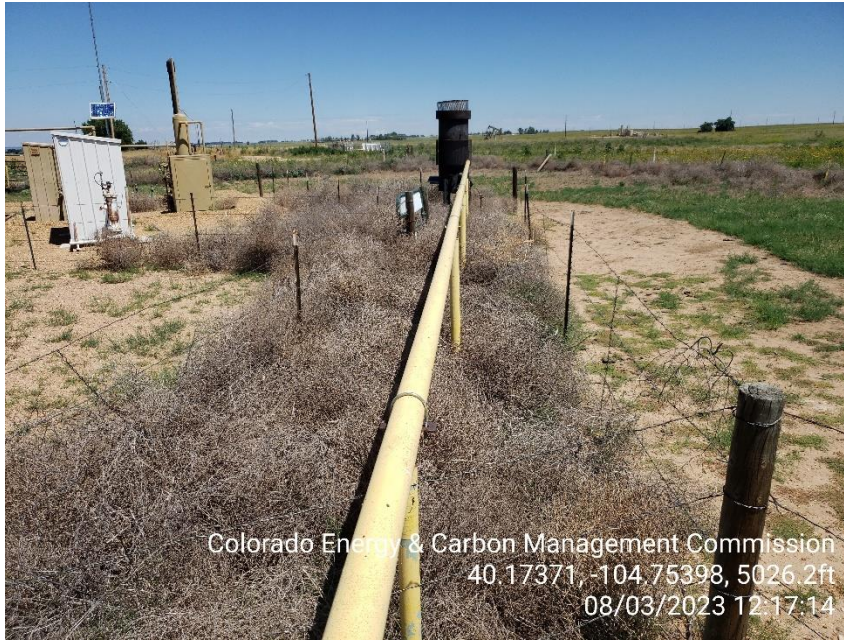
Photo 7 Tumble weeds accumulated around the ECD inside the fence.
