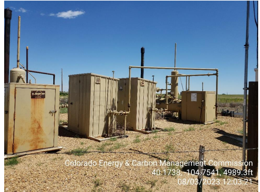
Photo 4 Horizontal Heated Separators, Gas Meter Run.
