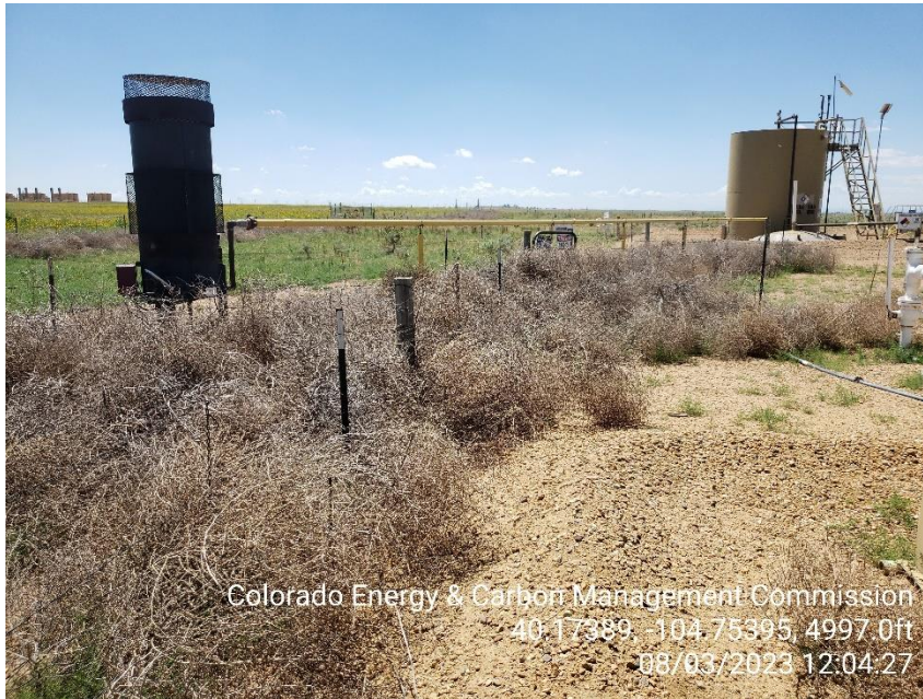
Photo 7 Tumble weeds accumulated around the ECD inside of fencing.
