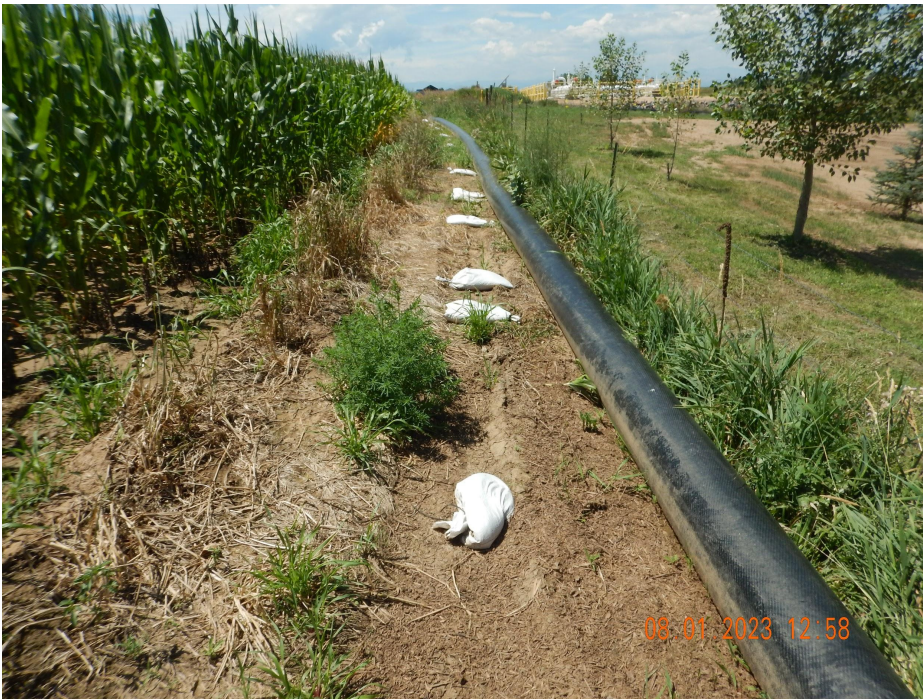
Photo 2. Photo illustrates the water line and sand bags, facing West. Sand bags were deployed by the Operator as a mitigation measure to allow irrigation tailwater to flow under the water line. Water line is no longer on sand bags.
