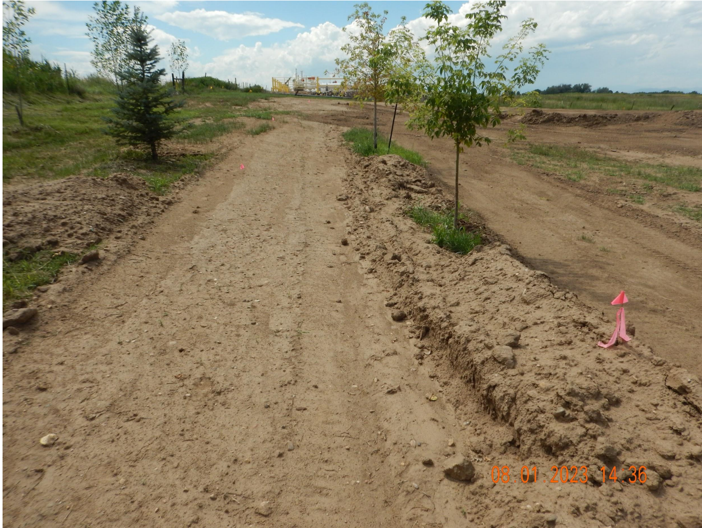
Photo 5. Photo illustrates a disturbed area that was planned for the installation of a BMP to mitigate irrigation tailwater run-on. Pink flags were placed by the Operator and yellow flags in the background were 811 locates. The temporary soil berm was constructed by the surface owner as a mitigation measure to protect their septic system.
