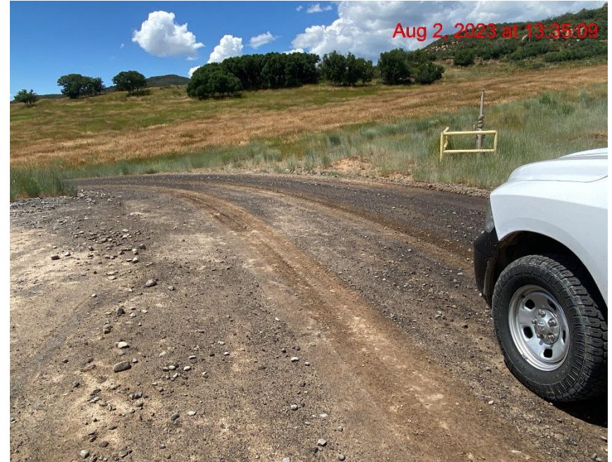
Insufficient Vehicle Tracking BMPs at Location Entrance/Exit – Photo #05418
