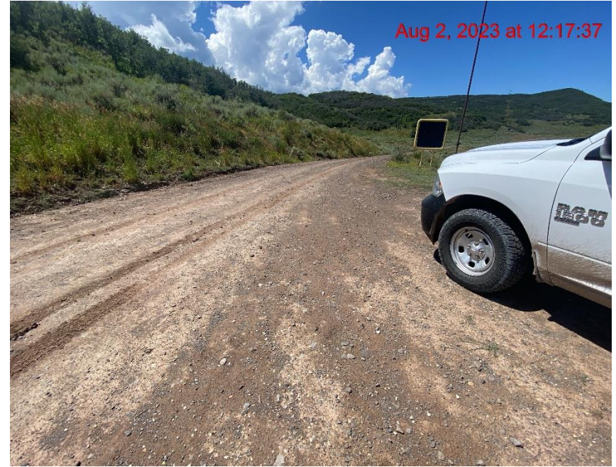
Insufficient Vehicle Tracking BMPs at Location Entrance/Exit – Photo #05388
