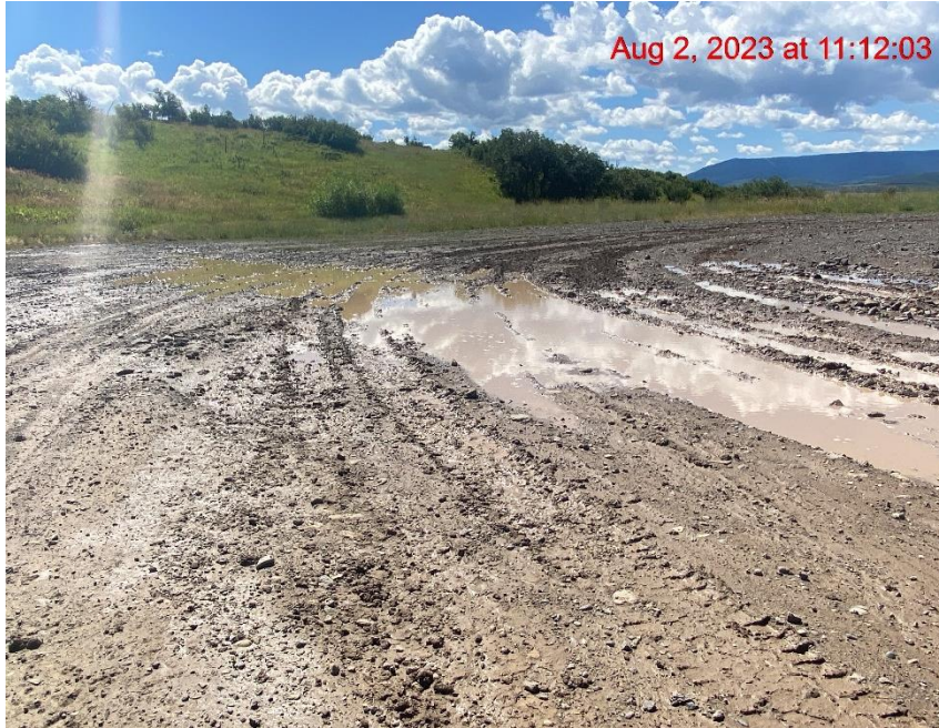
Location Lacks Stabilization – Photo #05363
