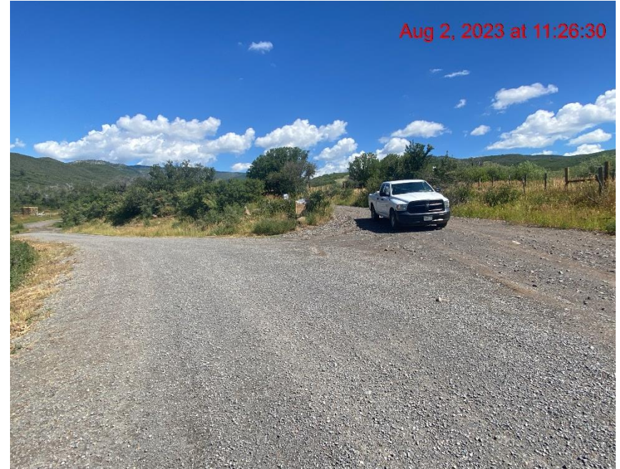
Insufficient Vehicle Tracking BMPs at Location Entrance/Exit – Photo #05367
