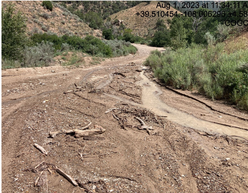
Access road washed out and debris
