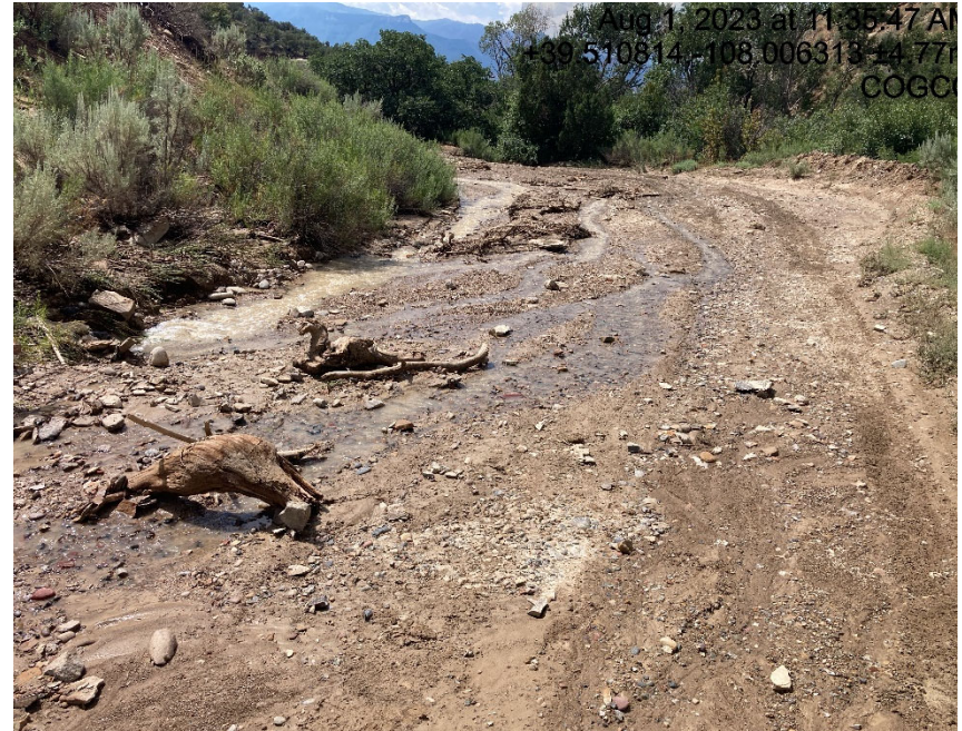
Access road washed out and debris
