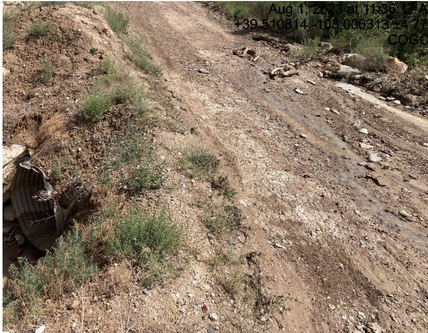
Culvert inlet is buried.
