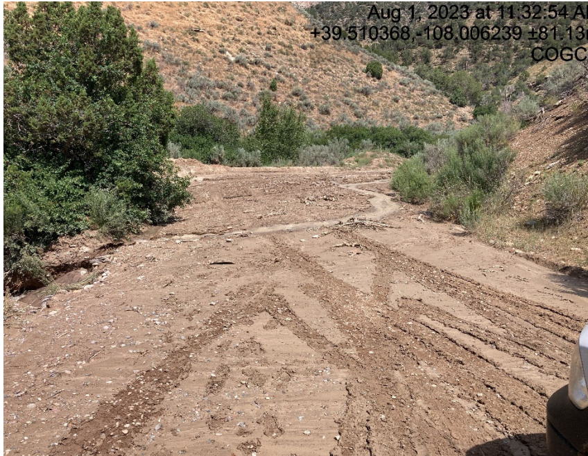
Access road washed out and debris
