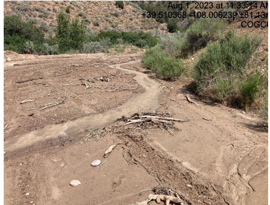
Access road washed out and debris
