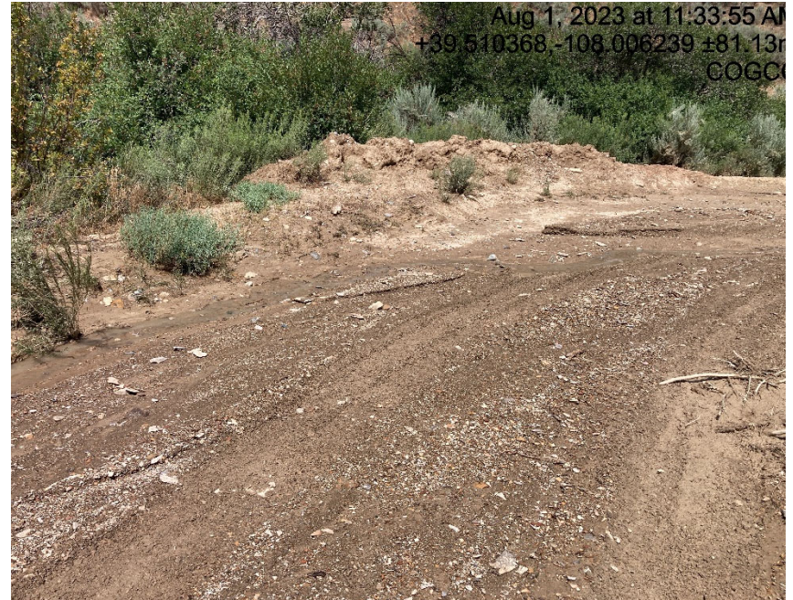
Access road washed out and debris
