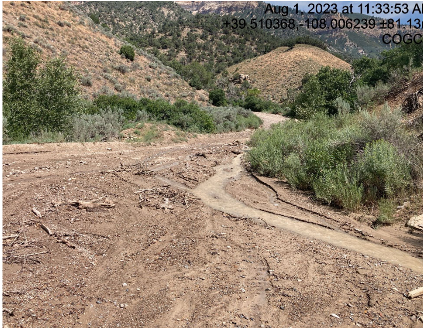
Access road washed out and debris
