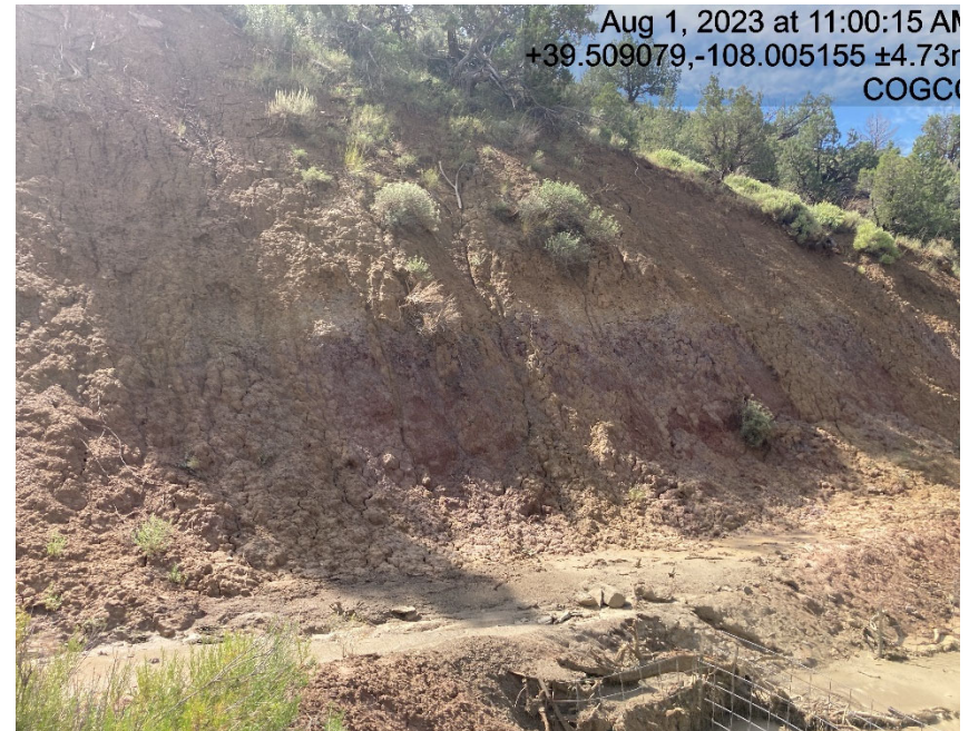
Cut slope lacks stabilization, riling and erosion
