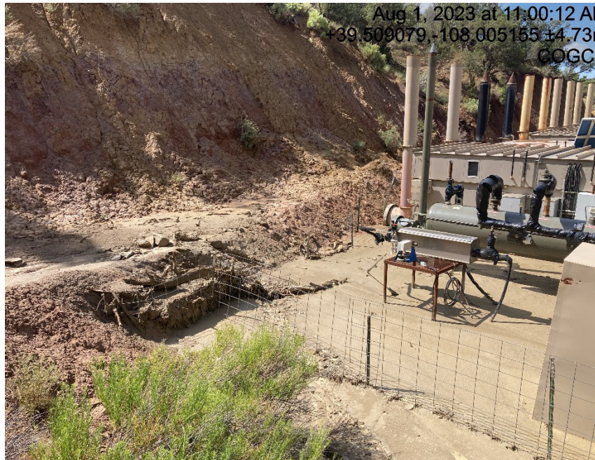
Cut slope lacks stabilization, riling and erosion. BMP's failing
