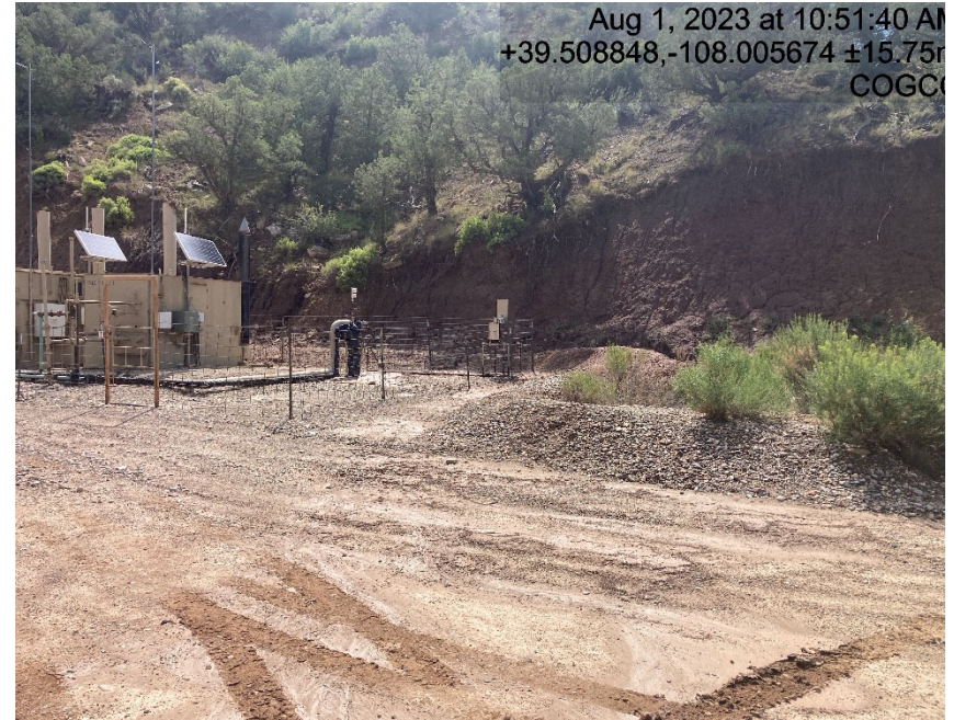
Cut slope sluffing off. Roots of vegetation is exposed.
