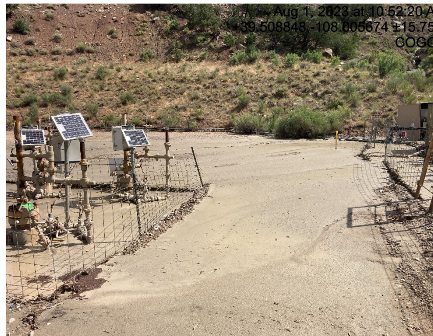
Location covered with mud. BMP's failing
