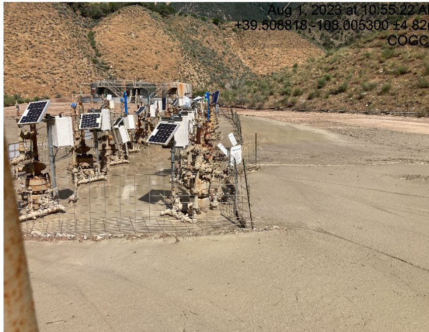
Location covered with mud. BMP's failing
