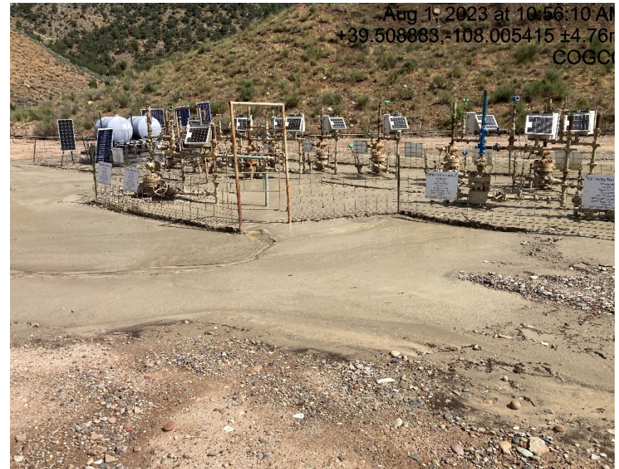
Location covered with mud. BMP's failing
