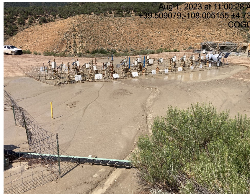
Location covered with mud. Storm water BMP's failing
