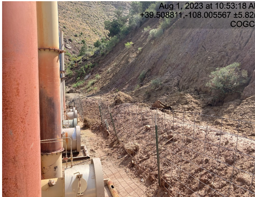
Cut slope lacks stabilization, riling and erosion
