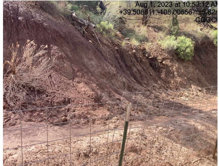
Cut slope lacks stabilization, riling and erosion
