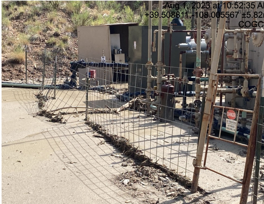
Location covered with mud. BMP's failing
