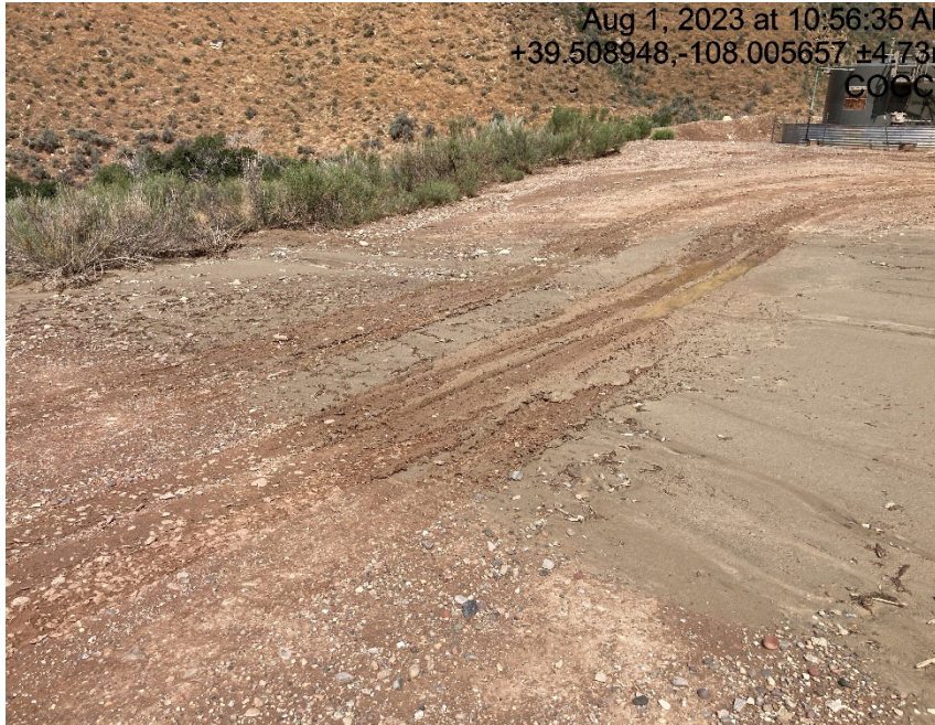
Vehicle has driven into mud which could lead to tracking issues
