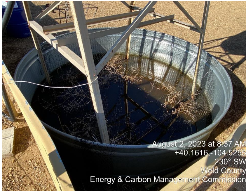
Inadequate Netting
