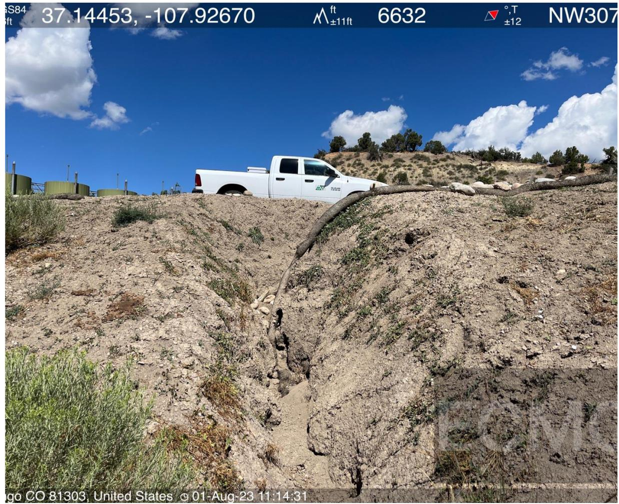
Photo #5. View of well location gully erosion.
