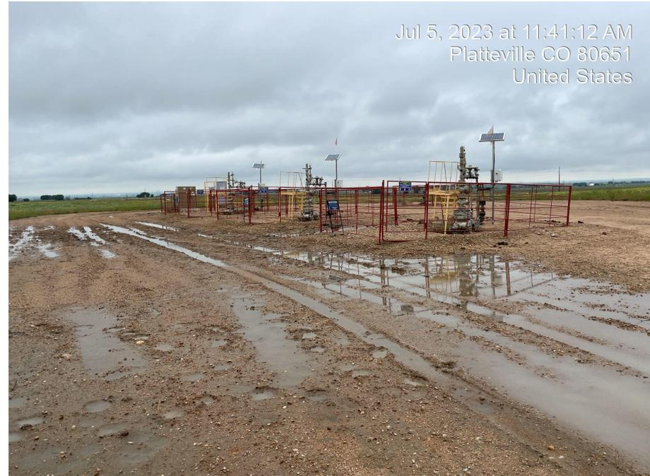
**Photo 5. Photo taken of stormwater erosion on access road.**
