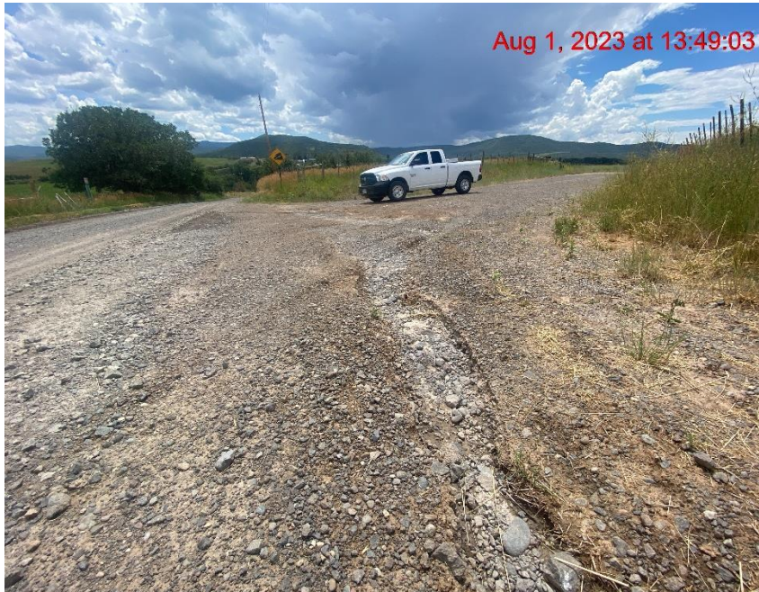
Rill Erosion Running Across Access Road – Photo #05305
