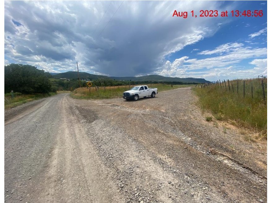
Insufficient Vehicle Tracking BMPs at Location Entrance/Exit – Photo #05304
