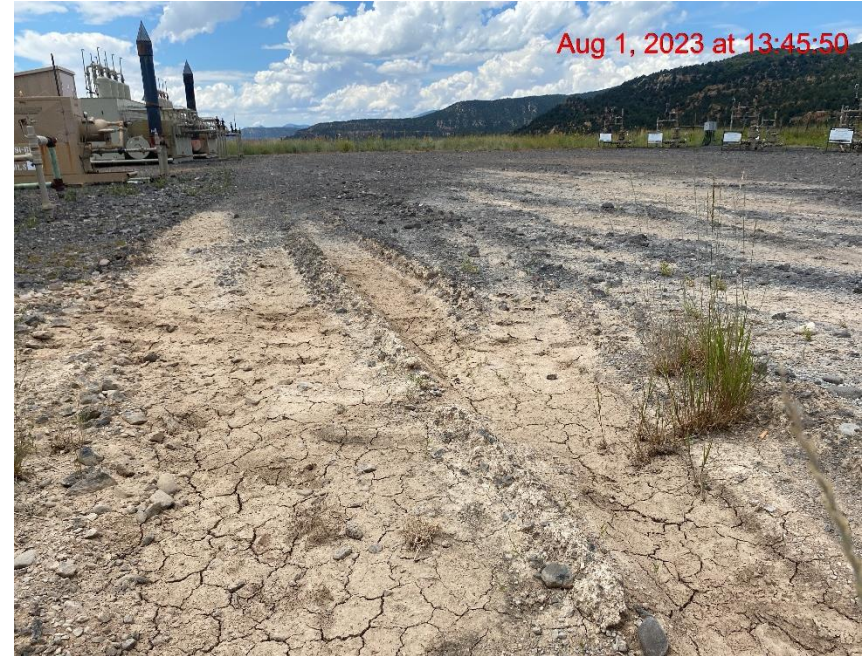
Location Lacks Stabilization – Photo #05300
