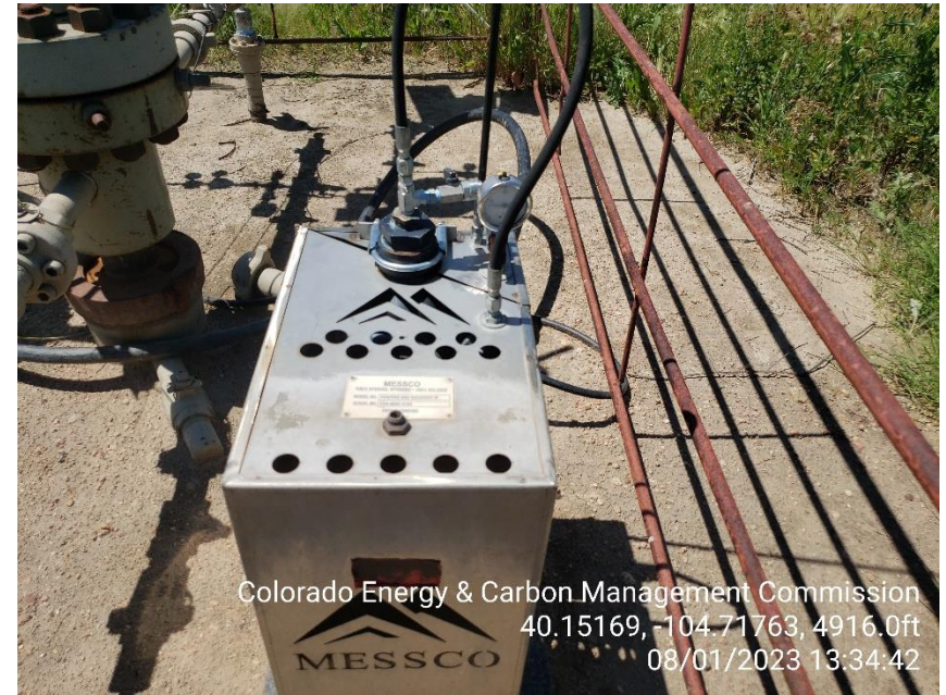
Photo 4 Fugitive Gas Combustion device.
