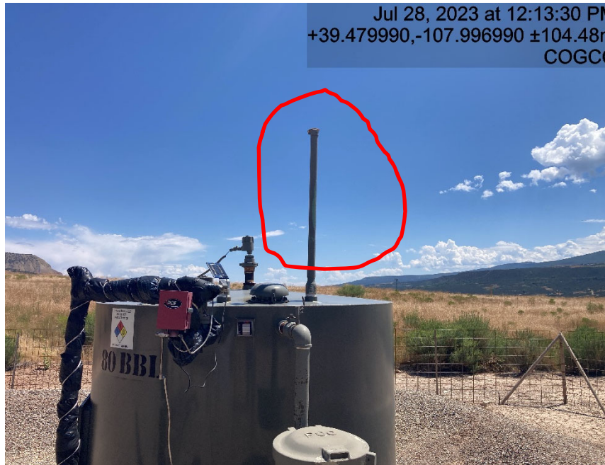
Line on top of tank open to atmosphere
