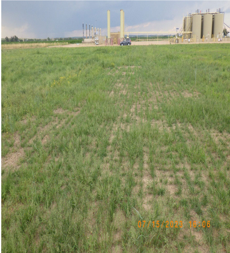
Photo 6. Overview photos of the well pad access road. Note: photo shows that operator has performed final reclamation activities with evidence of drill rows and straw crimped mulch. Site will remain in-process until uniform plant cover of at least 80% of the reference area is achieved.
