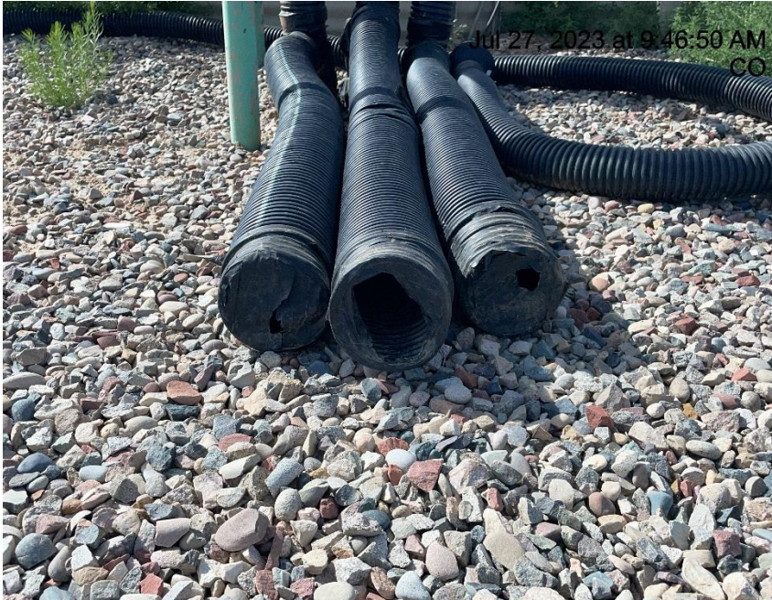
Photo # 3889 Flowline heating insulation open ended
