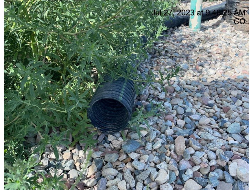
Photo # 3888 Flowline heating insulation open ended
