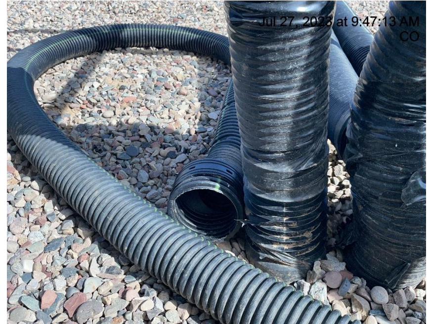
Photo # 3890 Flowline heating insulation open ended
