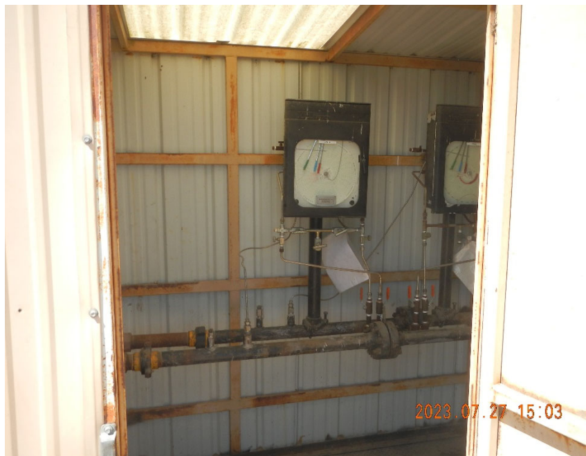
7. Gas Meter Run inside Meter Shed.
