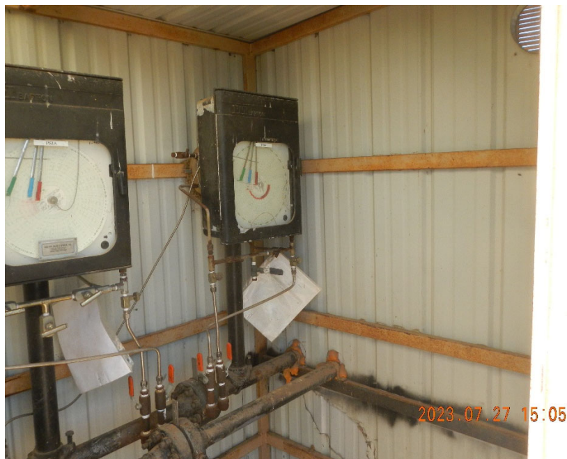
9. Remote Gas Meter Run inside Meter Shed.
