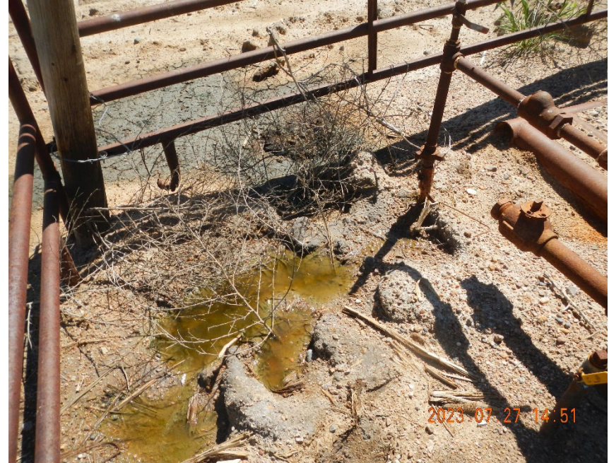
4. View of fluids inside SE corner of fencing. Soil is wet and saturated. Well is in active Pivot Irrigated Corn Field adding to moisture around well location.
