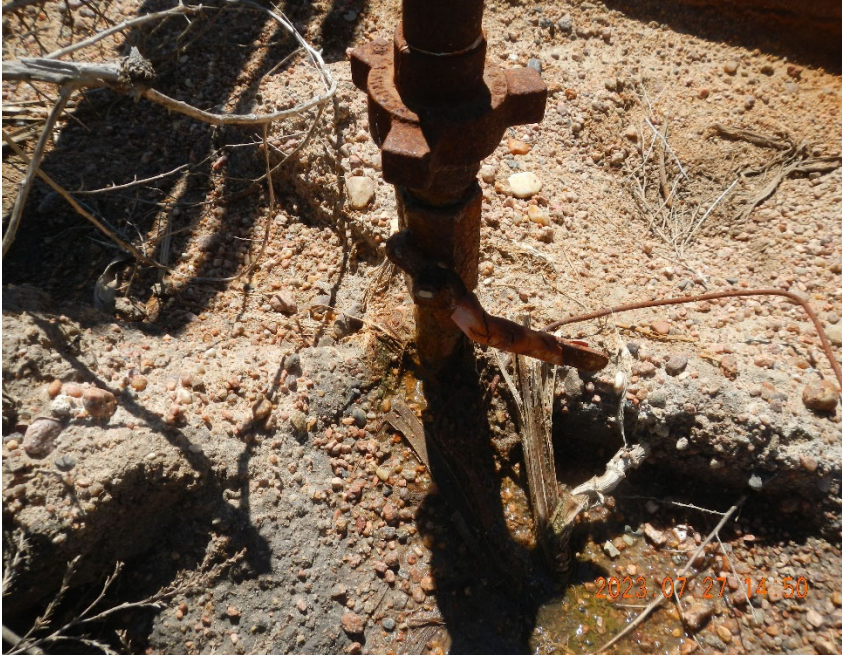
3. View of tubing produced water flowline with seep at hammer union threads.
