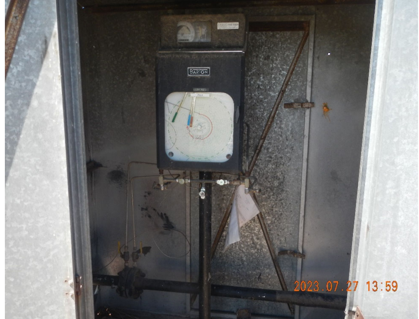
6. Gas Meter Run inside Meter Shed.
