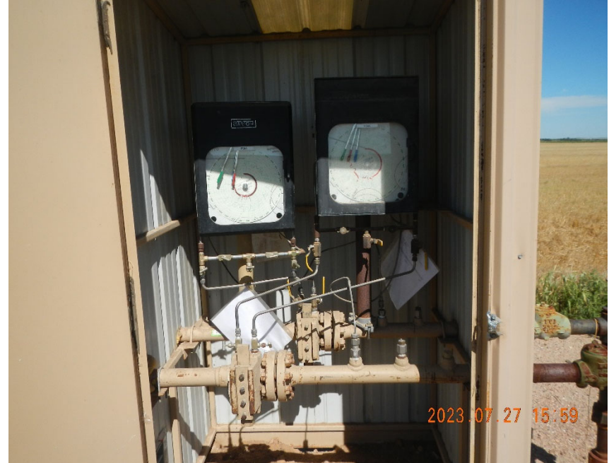
6. Gas Meter Run inside Meter Shed.
