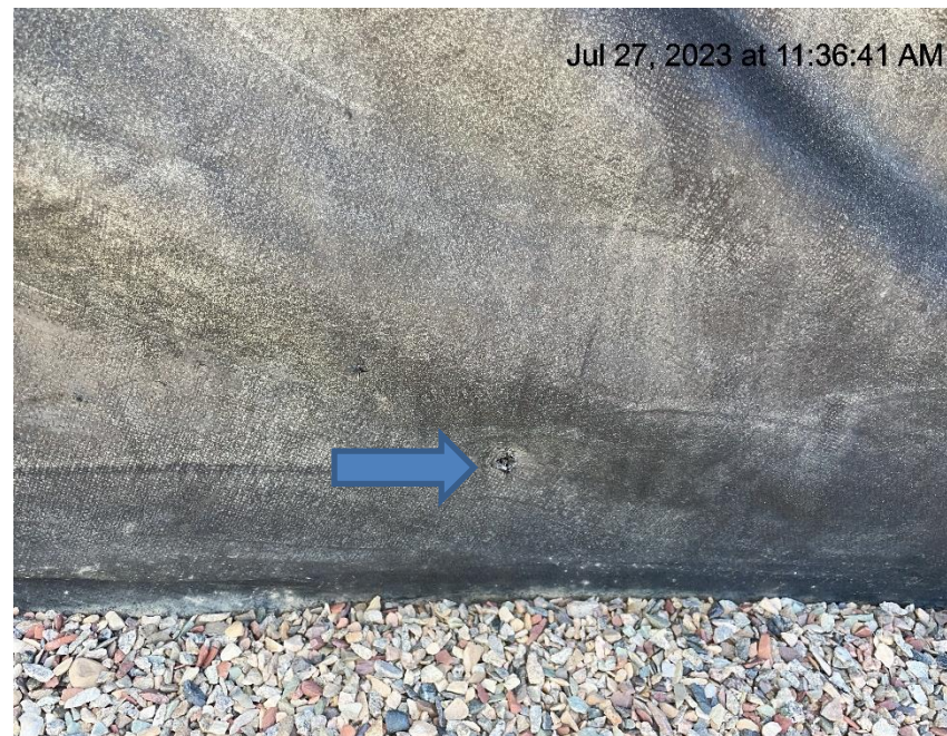
Photo # 4026 Secondary containment liner needs maintenance
