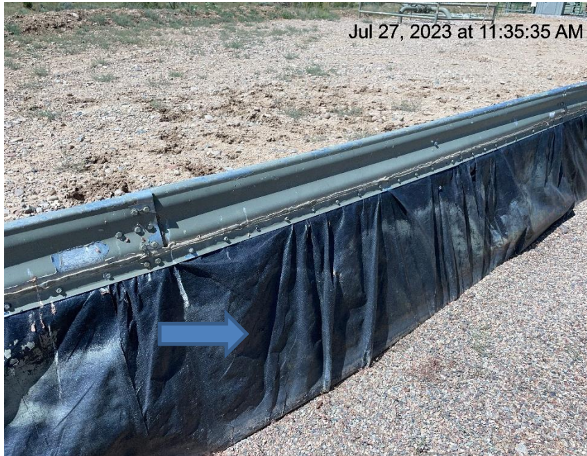
Photo # 4027 Secondary containment liner needs maintenance
