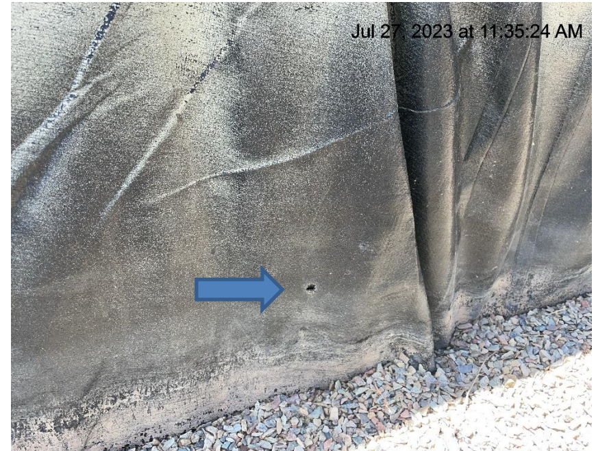
Photo # 4026 Secondary containment liner needs maintenance
