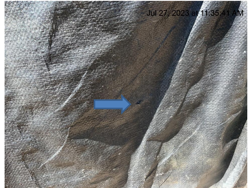
Photo # 4028 Secondary containment liner needs maintenance
