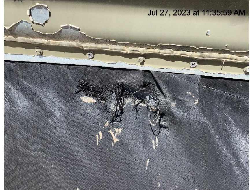
Photo # 4026 Secondary containment liner needs maintenance
