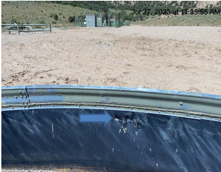
Photo # 4025 Secondary containment liner needs maintenance
