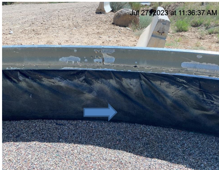
Photo # 4025 Secondary containment liner needs maintenance
