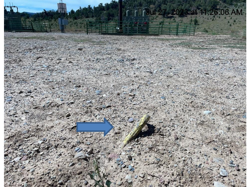
Photo # 4008 Same unmarked deadman from different angle
