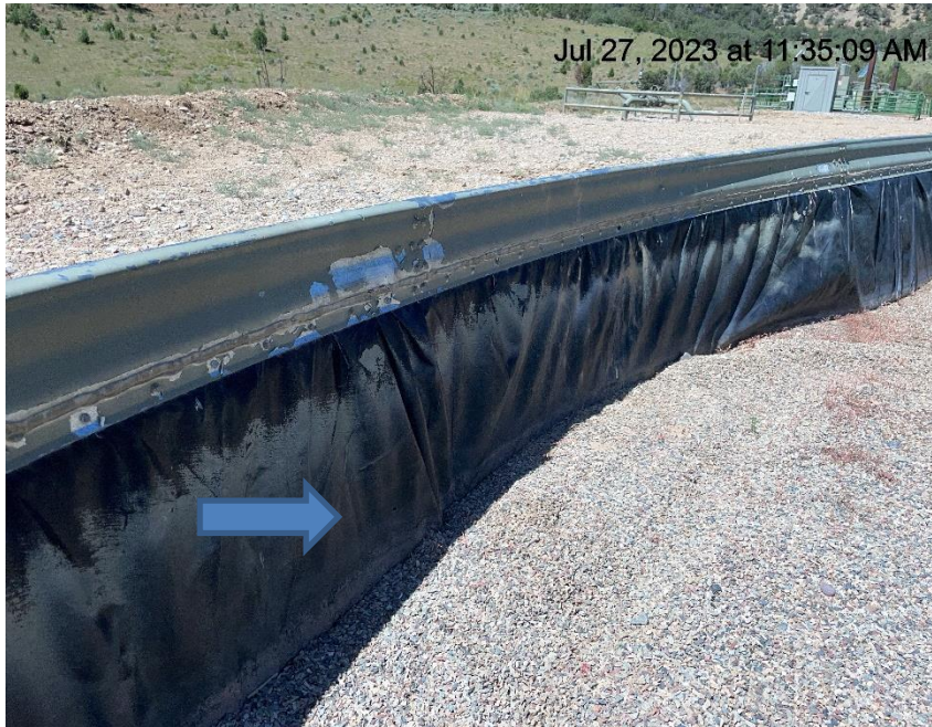
Photo # 4025 Secondary containment liner needs maintenance
